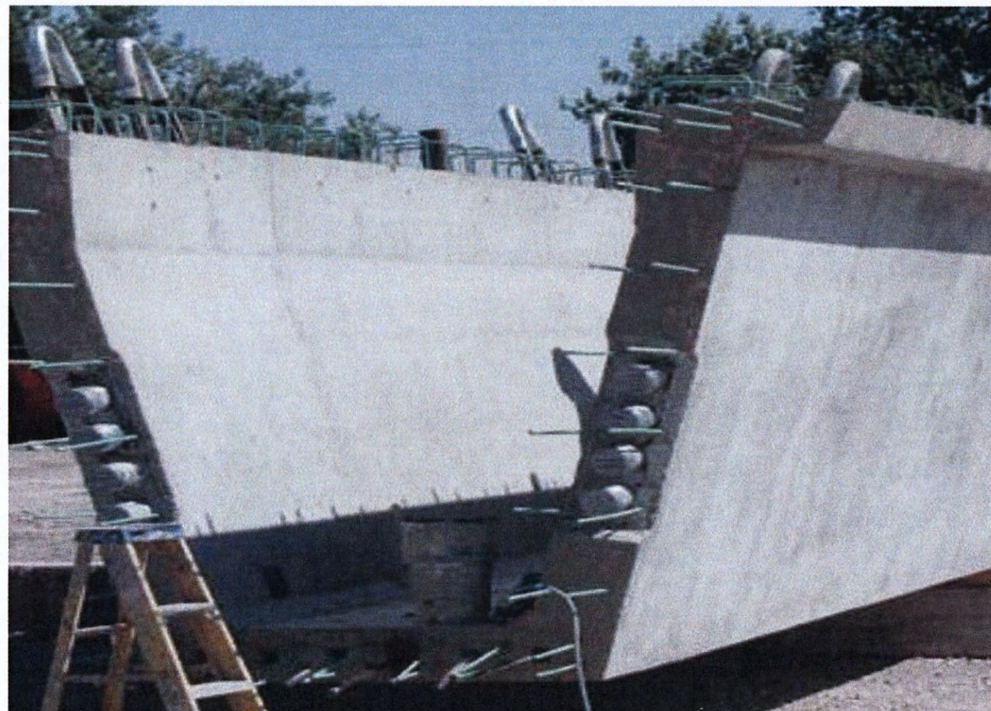
(b) Cross-section of U girders
