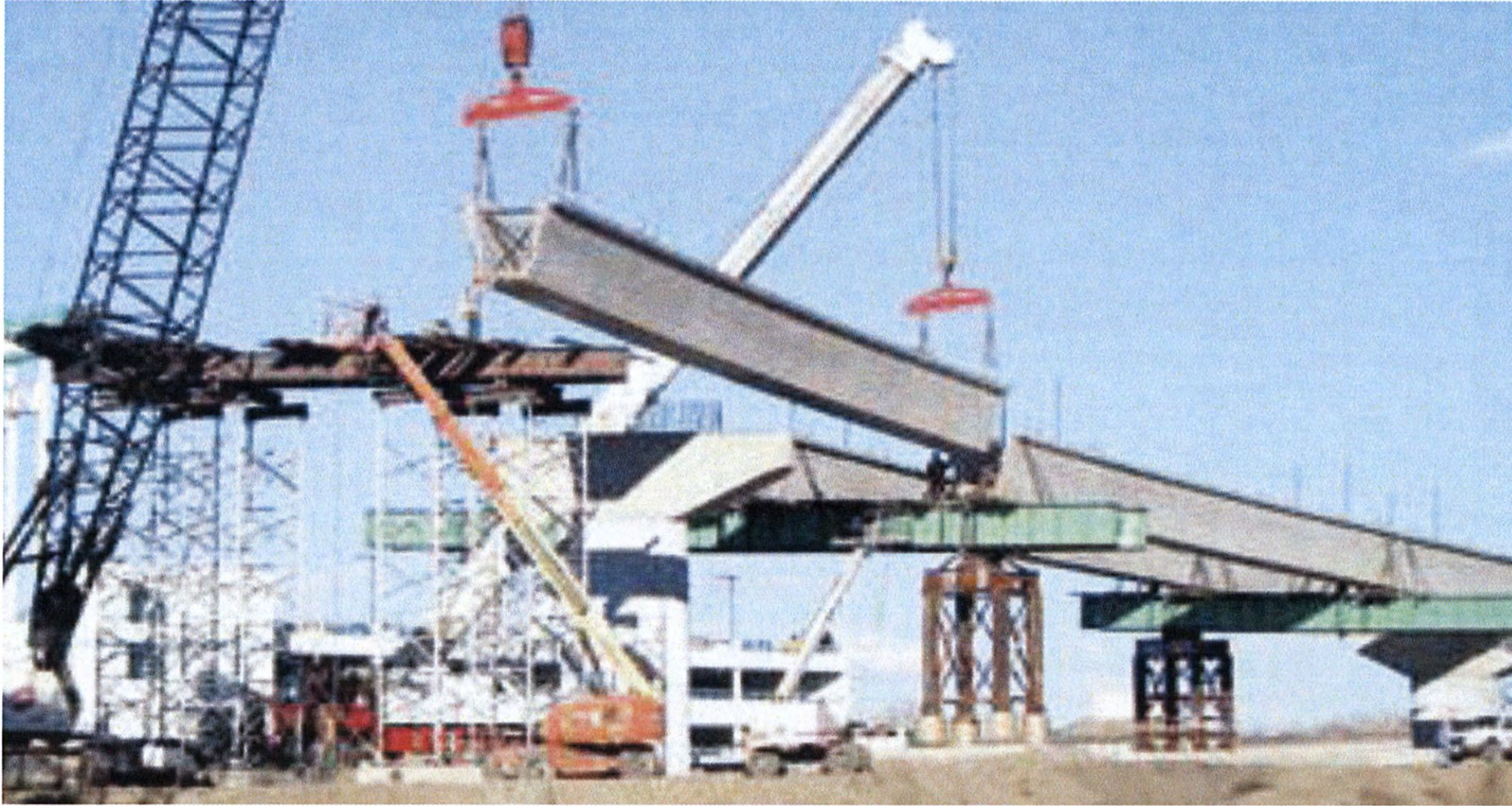
(a) Erection of U girders on site
