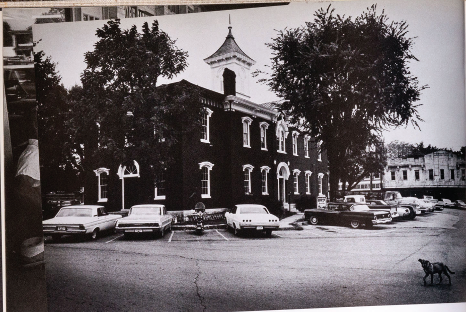
The sidewalks on all four sides of the Lynchburg Square are made of cement. But the people don't use them much. They want them to last.
