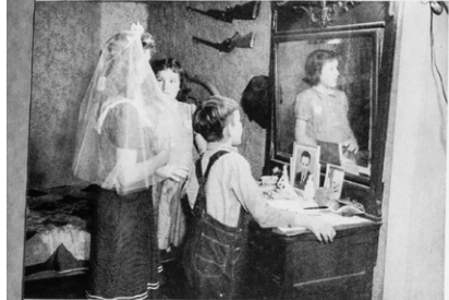
Hazel's wedding veil is previewed in bedroom by her sister Anna Ruth and brother "A. D." Hazel bought it in Middlesboro for $2.50, couldn't wait to take tag off before trying it on. Below: bride and groom, accompanied by Anna Ruth, walk 2 1/2 miles to the church (upper right). Groom carries wedding gown.
