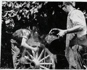
THE TIRED WHEEL IS IMMEDIATELY RUSHED to the cooling pit. The cooling shrinks the tire and makes it fit tight to the wheel.
