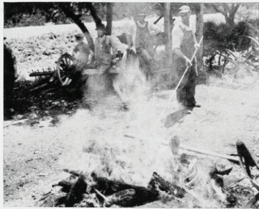
WAGON TIRES ARE STACKED IN A PILE and bits of old wooden rims are piled around them. A huge fire is lighted to heat and expand them.
