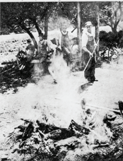
Completed iron tires are placed in an open fire to expand them so they can be mounted on waiting wheels.
