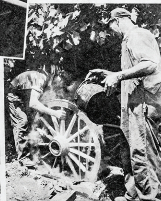
Once the hot tire is on, water is poured over it, to cool it and shrink it so that it can't come off. Wade Cline.
