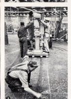
OLD PARTS ARE SALVAGED for new machines at Willow Run. A drill press is pulled in by tractor (1). It passes a pile of parts salvaged from the Livonia shambles (2). Larry Touzeau, a veteran toolmaker, consults blueprint (3) as he
