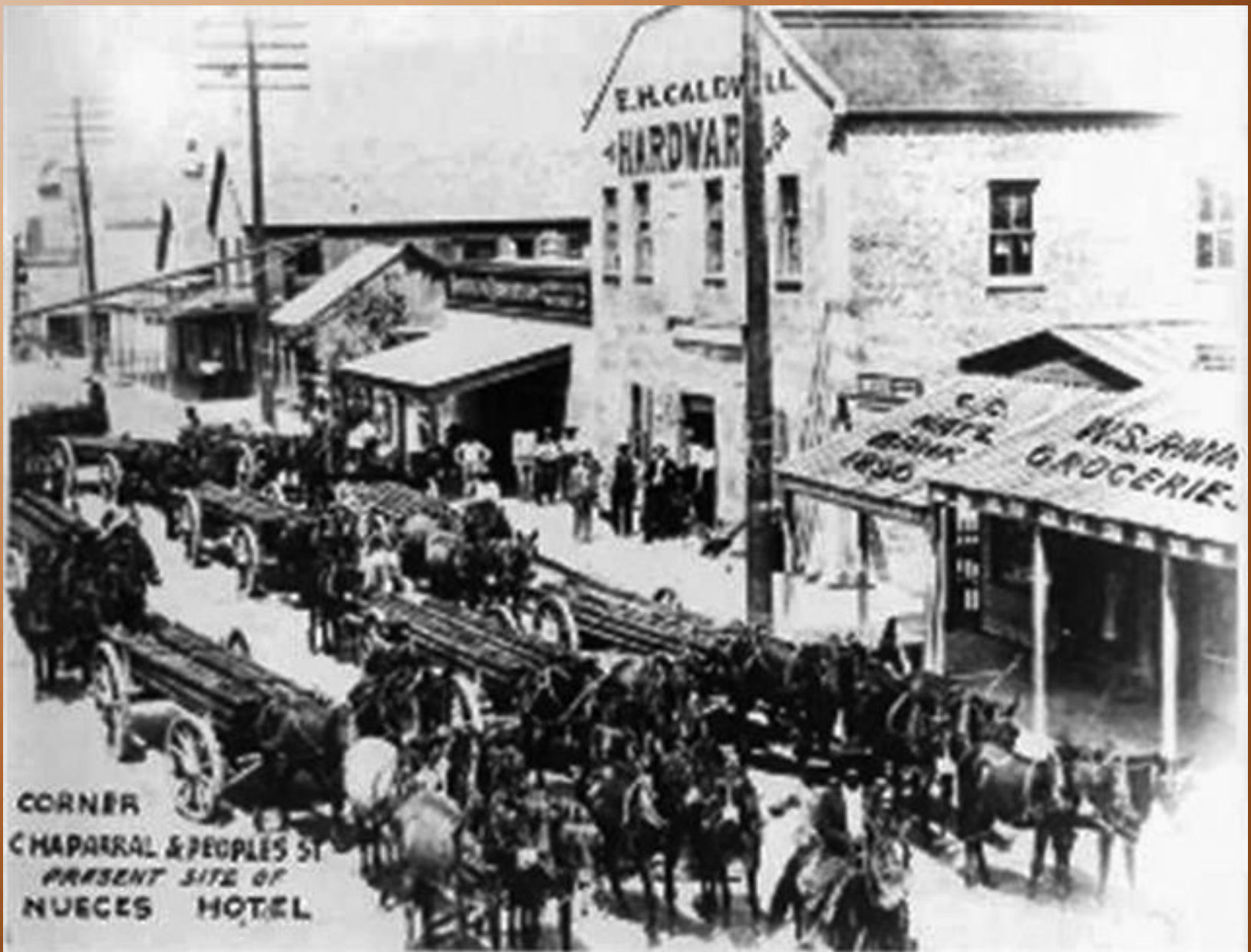
Wagons with pipe heading for the King Ranch to drill water for artesian wells in 1899
