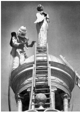
Key: 6-1-2.5ii Sandblasting.tif
