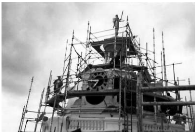
Key: 6-1-3 Timeline - scaffolding.tif
