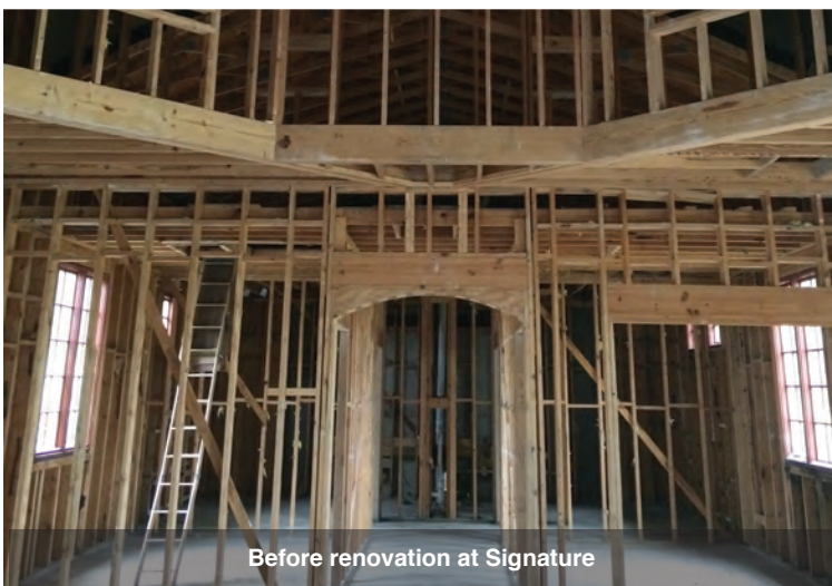
Before renovation at Signature
