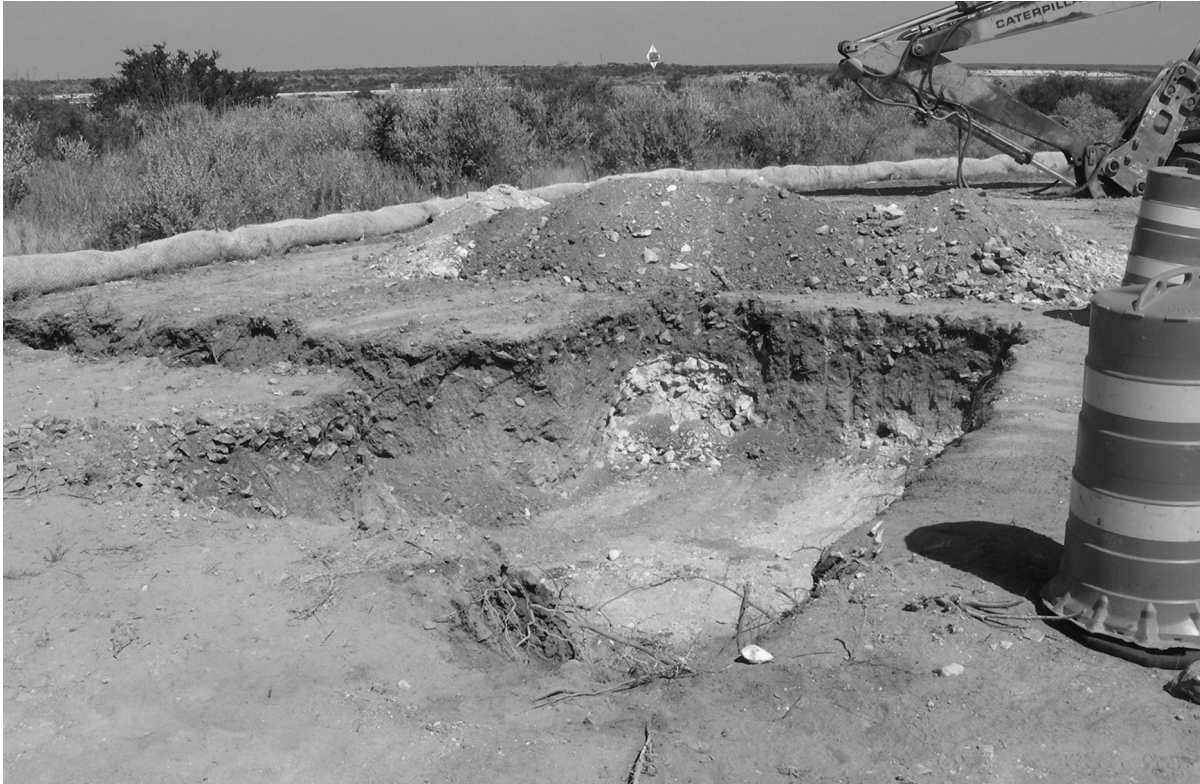
Figure 1. Backhoe excavation at previously unknown site 41VV1991, the Lost Midden site.
