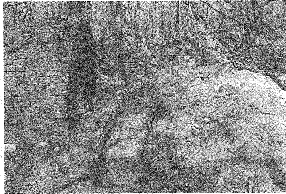
Figure 7. Arched Brick Entry of Flue Chimney. On the left can be seen the arched brick dome of the entrance to the flue chimney. The flue took a right turn to enter the chimney from its path under the kettles seen on the right.
