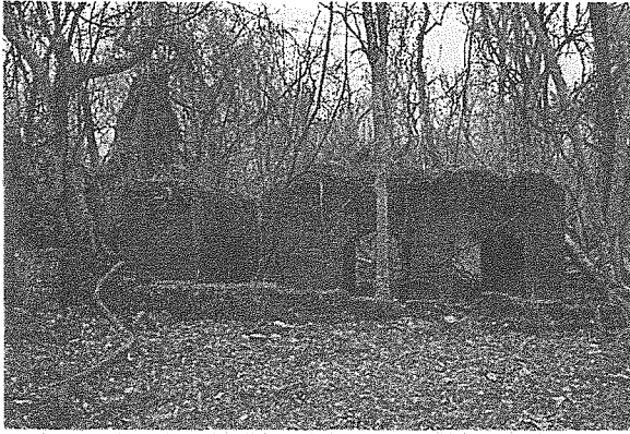
Figure 4. Brick Foundations at Osceola that supported the Engine and Cane Crushers.
