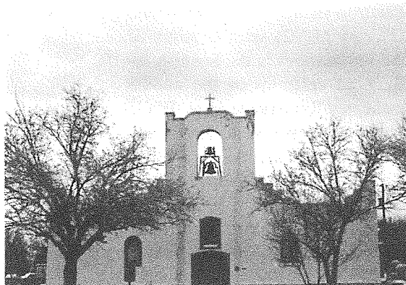
Figure 13. Socorro Mission, stepfret parapet design.
