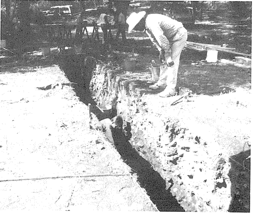
Figure 6. W110 Units Nearing the Completion of the Labor Day Excavations. Looking to the South.
