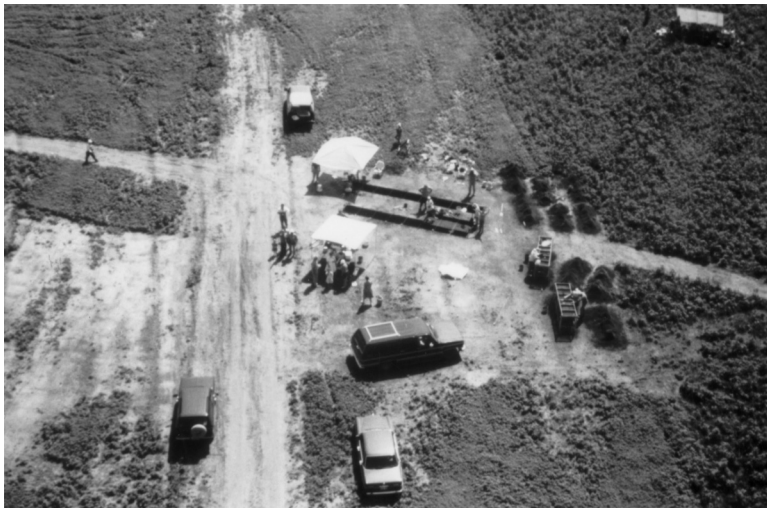
Figure 16. Aerial view of the Block III excavations in June 1991.
