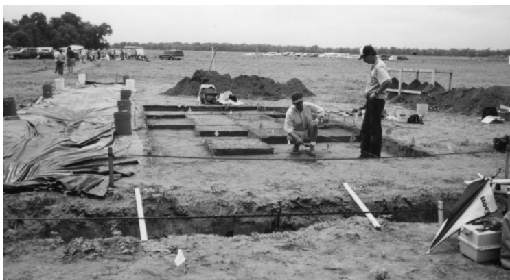
Figure 8. Block II excavations, looking south.
