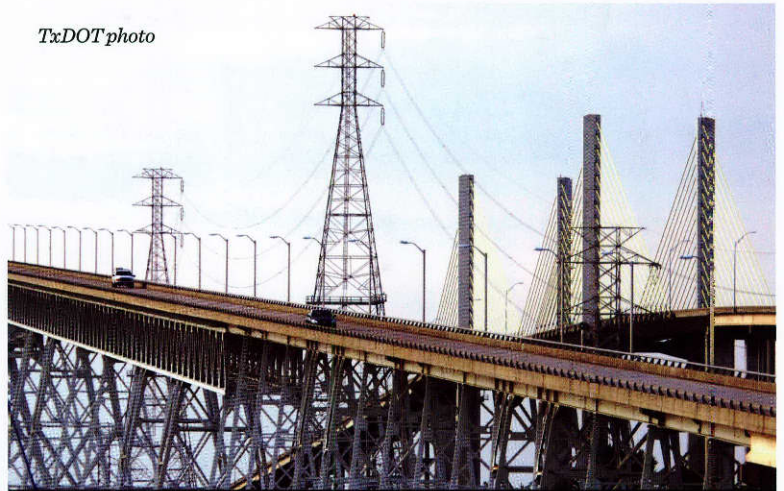
Built in 1938, the Rainbow Bridge (foreground) between Bridge City and Port Arthur is the steepest cantilevered through-truss bridge in Texas, spanning 176 feet above and 630 feet across the Neches River. The Veterans Memorial cable-stayed bridge next to it opened in 1990 and carries traffic in one direction.
