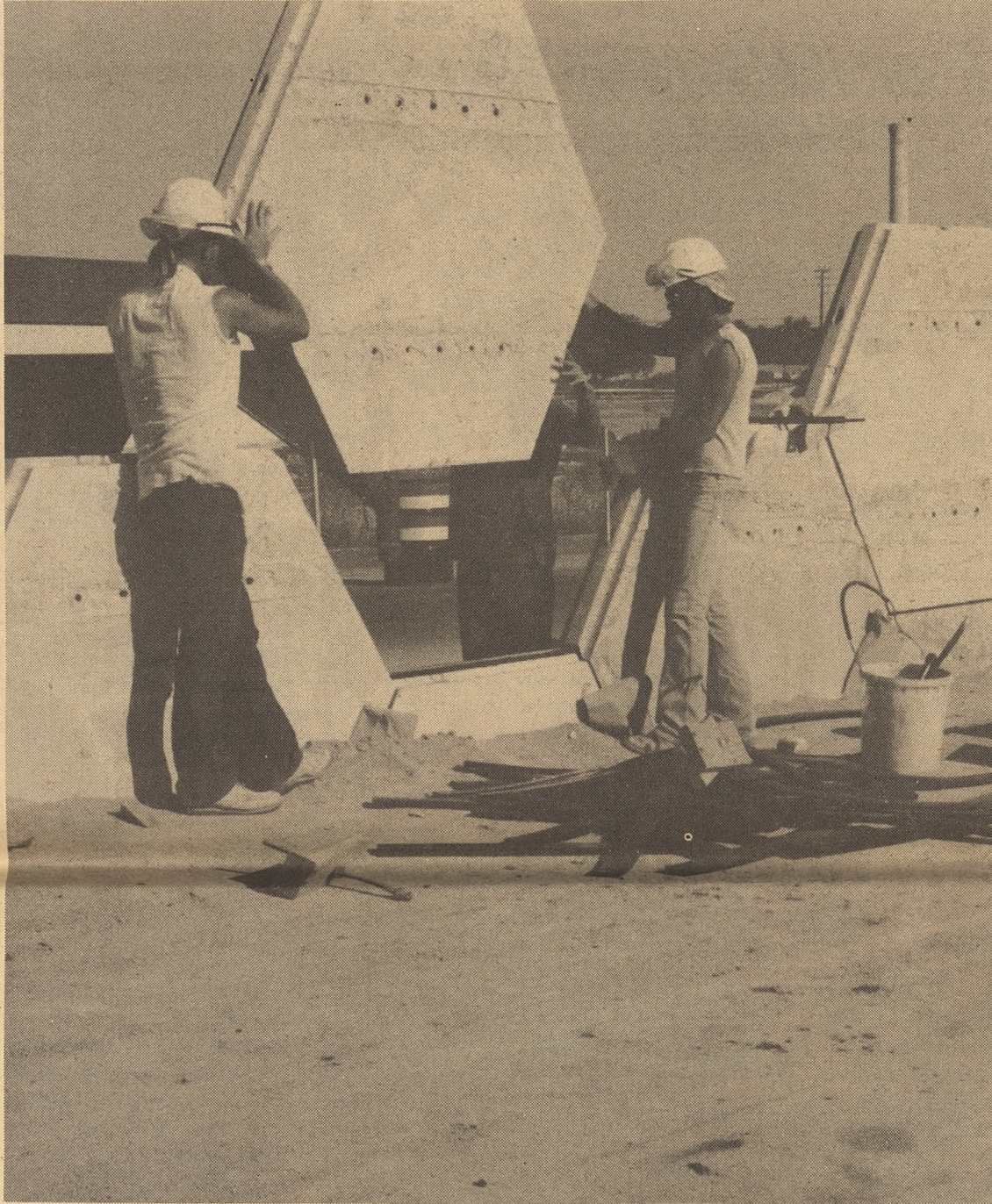
Construction workers guide the panels into place.
