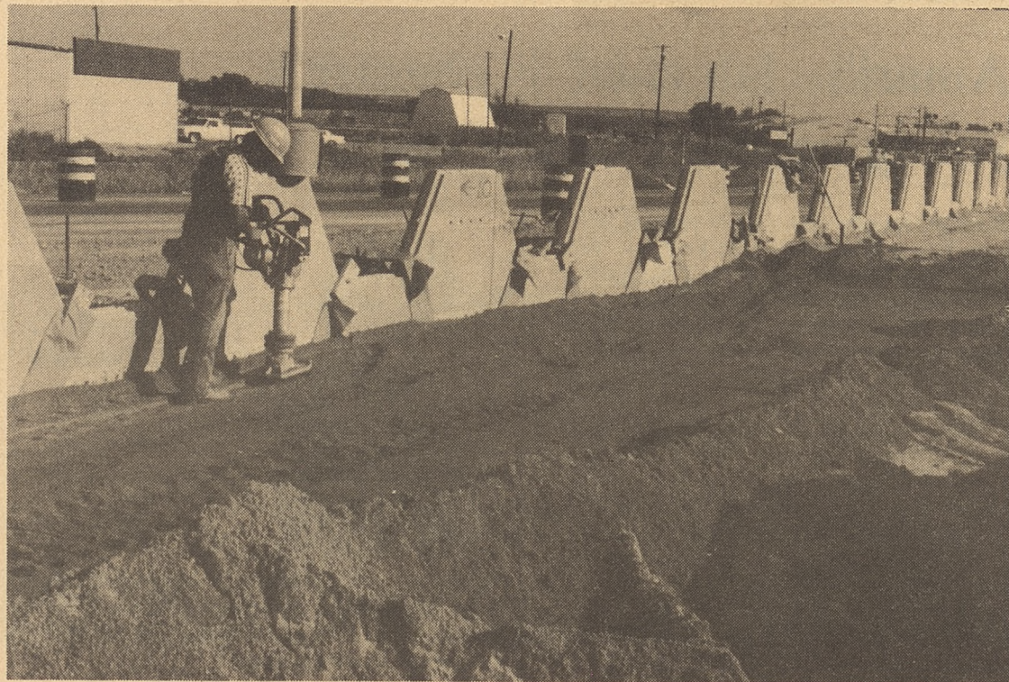
Backfill is compacted over the reinforcing mesh.
