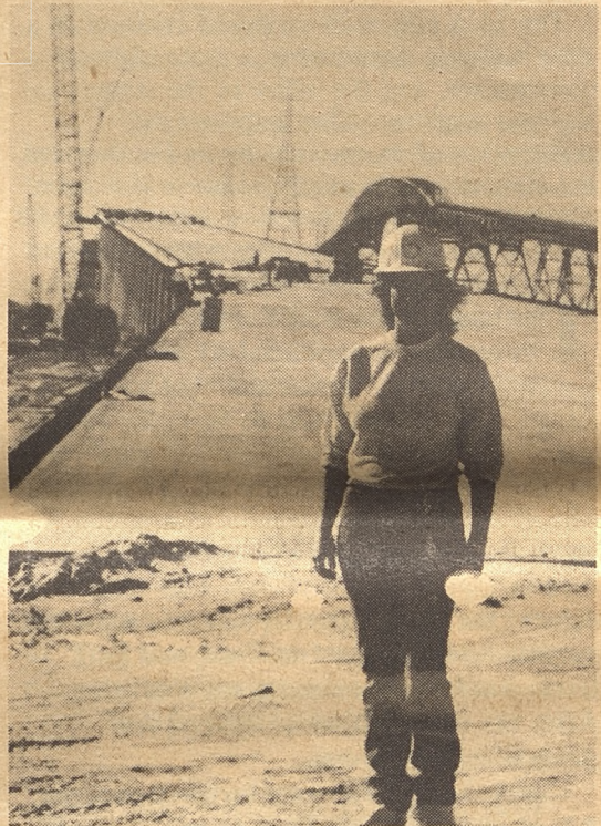
Charlotte Warner is project engineer for the $26 million new Rainbow Bridge in the Beaumont District. The new, cable-stayed bridge will be 9,440 feet long. (Photo by Nancy Stout)
