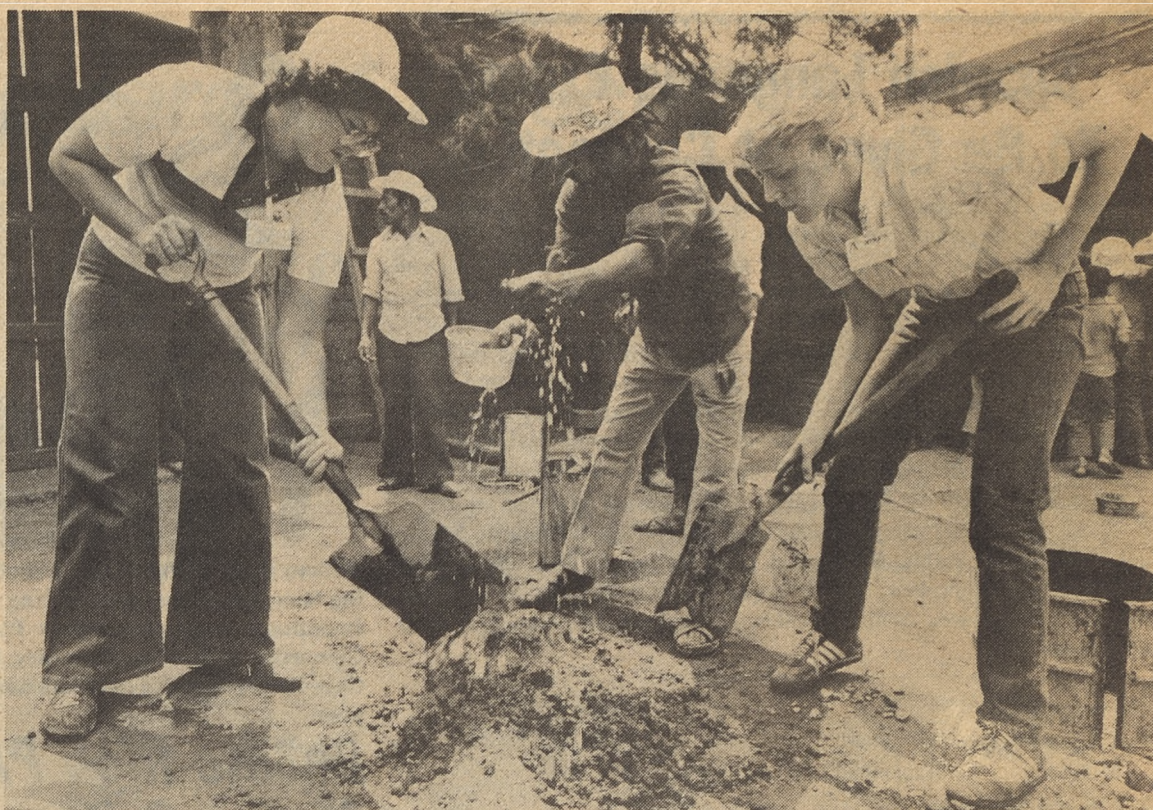
AMIGOS volunteers mix cement for the latrine construction in Mexico.
