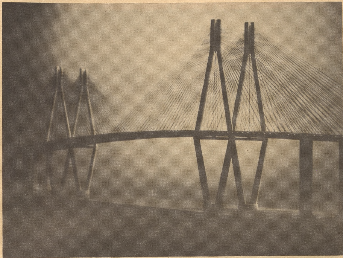
Baytown bridge will feature double-diamond design and longest cable-stayed span in the nation, at 1,250 feet. Construction of the steel structure is expected to continue for five years.
