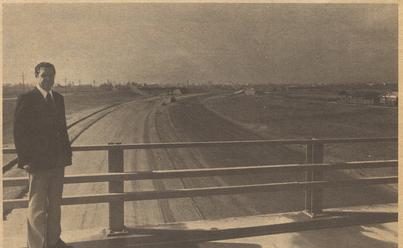
Lubbock Resident Engineer Volney Chetty has been named Engineer of the Year by the South Plains Chapter of the Texas Society of Professional Engineers. Chetty has been actively involved in the work on IH 27 in Lubbock.
