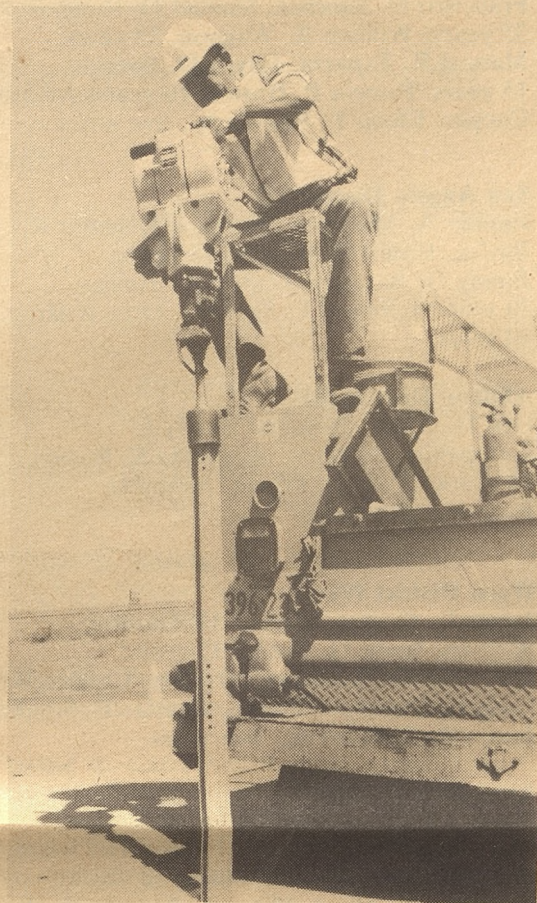
With the Pionjar, one person can drive a signpost from atop the rear of a pickup truck.
