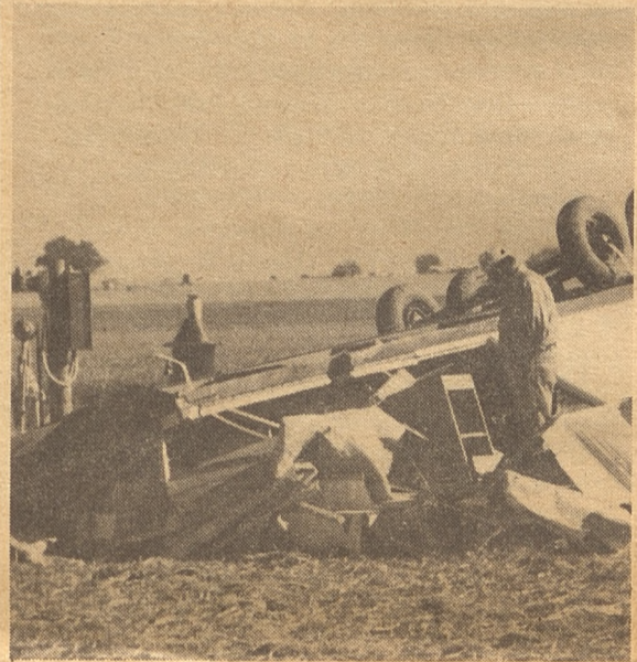
Raul Martinez, inspector in the Plainview residency, looks over what's left of the field office.
