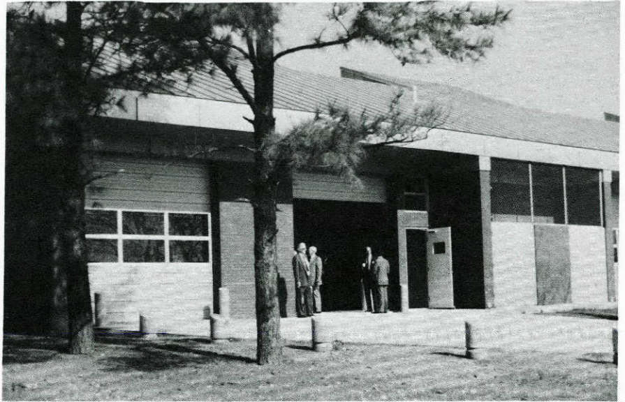
NEW VOCATIONAL BUILDING at Gainesville State School was the site of an open house March 13. This entrance is actually at the rear of the building, where the open house event was held.
