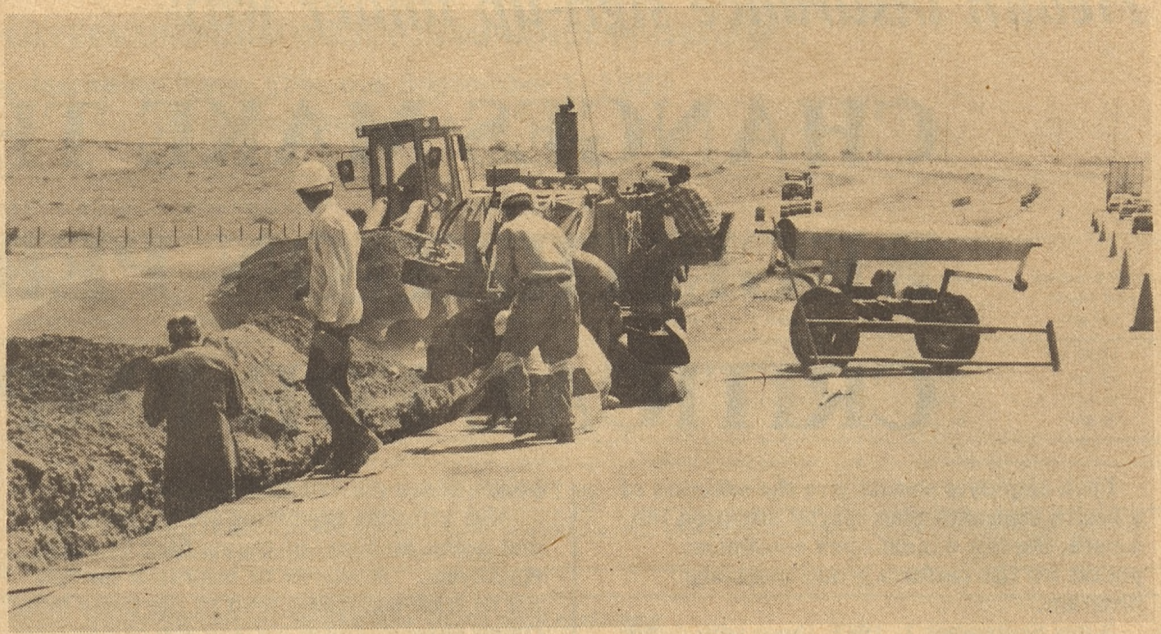
El Paso Sand Products Company crew places moisture barrier.
