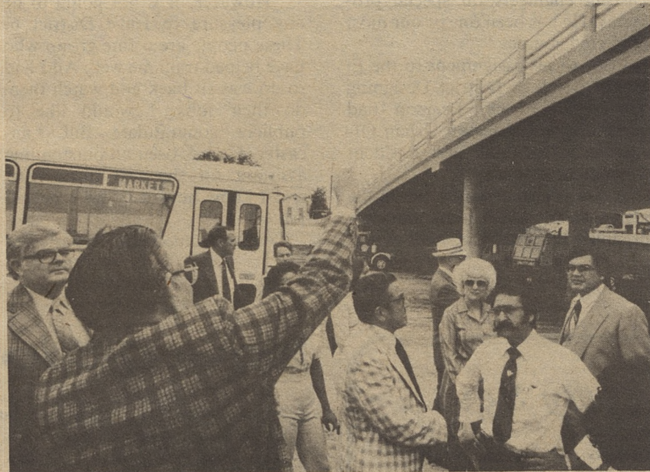
Laredo officials got a tour of the IH 35 project riding one of El Metro's new buses.
