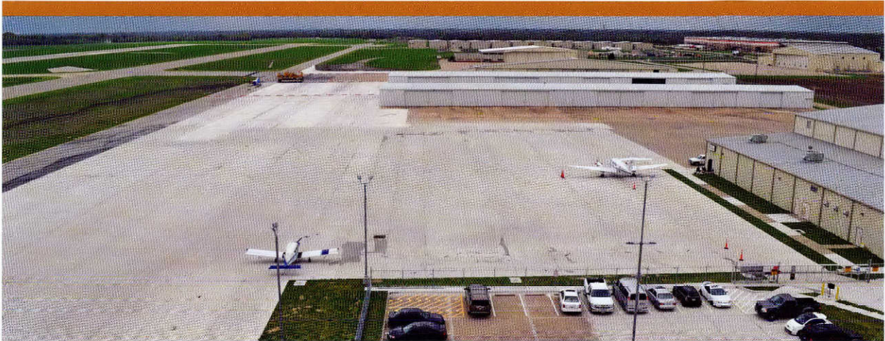
The relocated automobile parking lot and expanded terminal area apron at McKinney National Airport.
