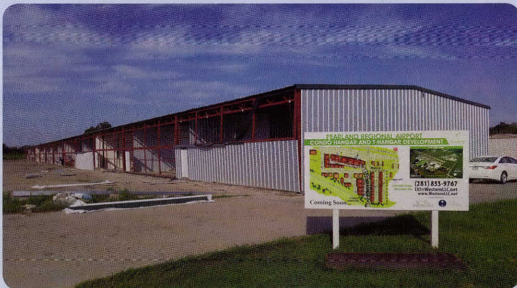
Hangars under construction at Pearland Regional Airport.
