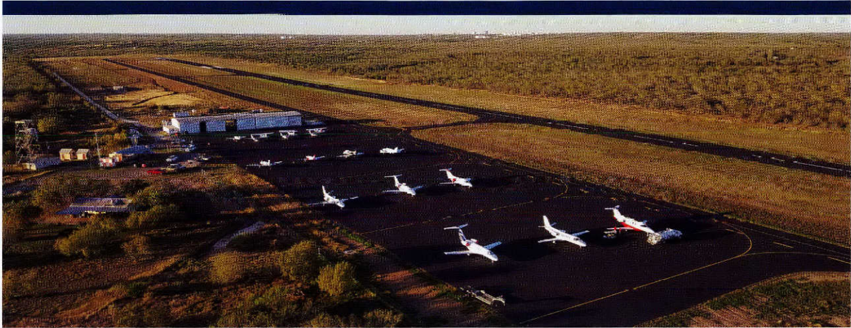
Aerial view of the completed runway 13-31, extended taxiway and expanded apron at Cotulla-LaSalle County Airport.
