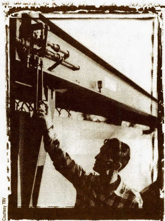
A Lufkin employee works on prestressed concrete operations.
