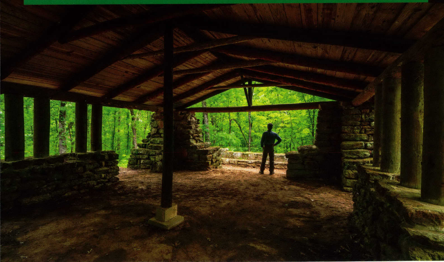
The Civilian Conservation Corps built this stone-and-timber pavilion at Caddo Lake State Park during the Great Depression.
