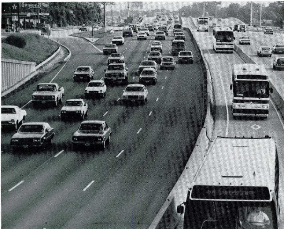
High occupancy vehicle (HOV) lanes on a number of urban freeways ease congestion by promoting the use of commuter buses, car pools, and van pools.
