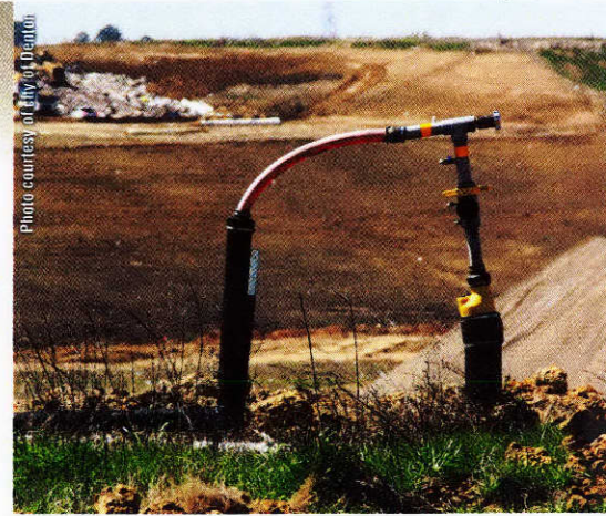
Harvesting methane for energy is important to the Denton landfill. An enhanced leachate recirculation system takes the liquid that percolates out of the packed trash in the landfill and pumps it back through the waste to help break down natural materials. The result of this is an increase in methane gas production, which is a natural byproduct.
