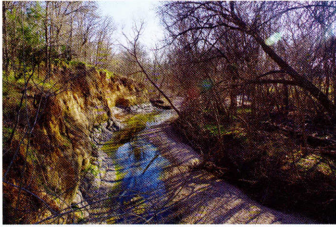
Figure 3.1 - Erosion on Williamson Creek. Image courtesy of Johnnie Smith.
