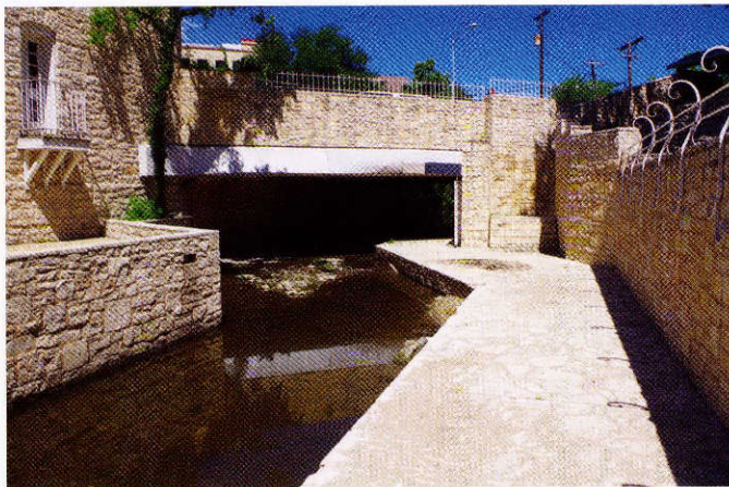
Figure 8.8 - Waller Creek in downtown Austin, Texas, is a great example of a channelized urban stream.. Image courtesy of Johnnie Smith.
