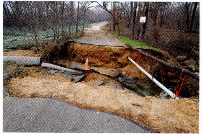
Figure 7.8 - Floods in Bastrop followed the fires. Rain soaked soils laid bare by the fire quickly eroded and washed out waterways. Here the earthen dam was washed out on Copperas Creek, draining the lake in Bastrop State Park. Image courtesy of TPWD.
