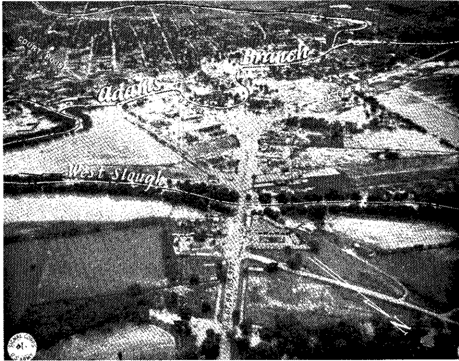
FLOOD ON ADAMS BRANCH-1945 AT BROWNWOOD, TEXAS
