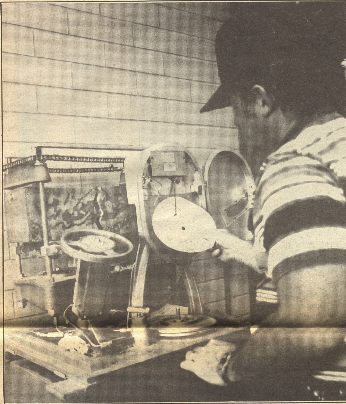
William Beaver, of the Austin District Lab, tests the strength of a mini beam from concrete being used at a San Marcos project. (Photo by Harvie Jordan, ABC)
