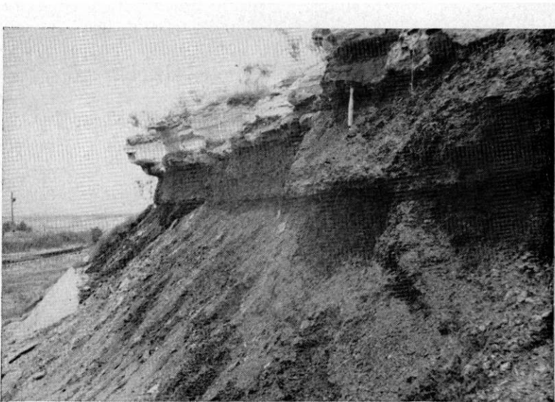
Figure 4.—Austin-Eagle Ford contact, quarry of the Trinity Portland Cement Company.
