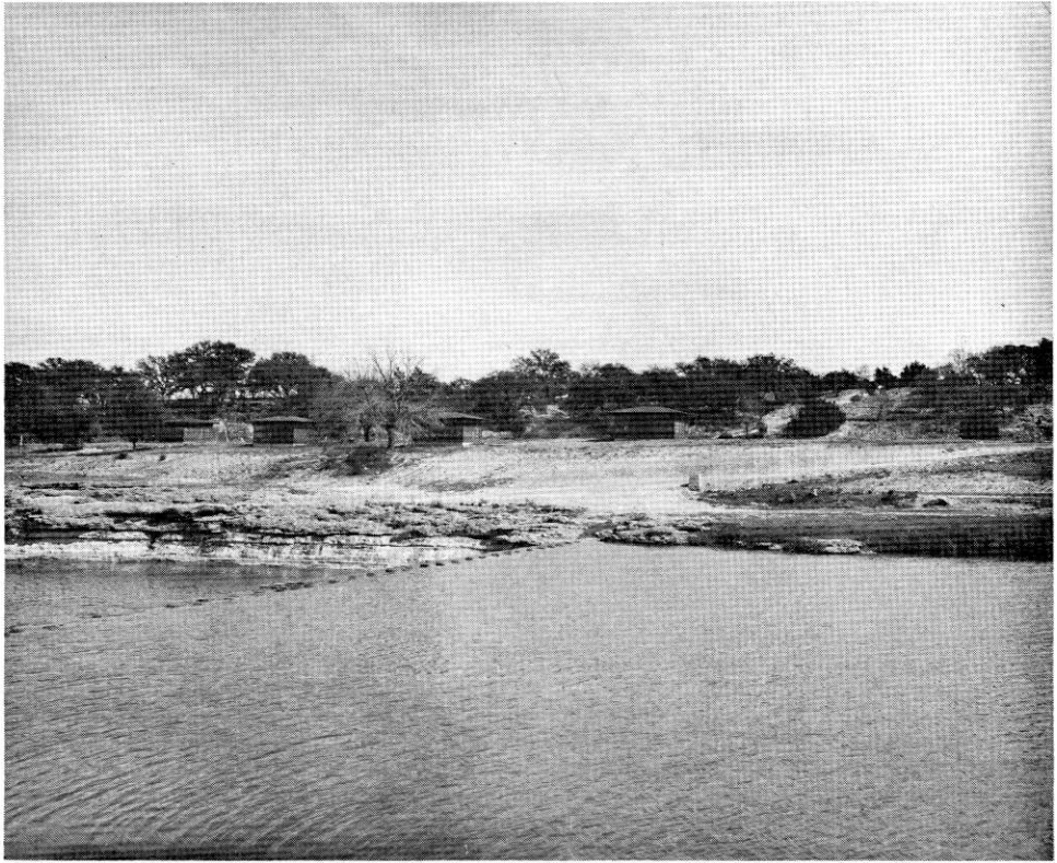
FIG. 29. Hard and soft rock layers in the Glen Rose Limestone at Blanco State Park. The limestone ledge near water level is sufficiently resistant to support the low-water dam. The screened shelters are on a thin resistant ledge that underlies a gently sloping surface. The top of the ridge is also capped by resistant limestone. The slopes in front and to rear of the shelters are underlain by less resistant marl. Stairstep topography similar to this profile is common in areas underlain by the Glen Rose. (Photograph by Texas Parks and Wildlife Department.)
