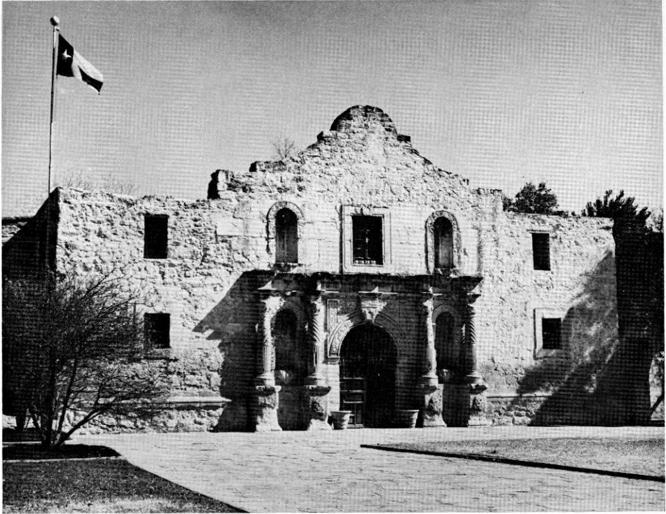
FIG. 23. The Alamo. The walls of the Alamo are now plastered and most of the rock masonry is covered. The rocks used in constructing the walls are mostly roughly hewn blocks probably from the Austin Group (table 1). Location of the original quarry is not known, but the rock looks like that now exposed in the old quarries within Brackenridge Park. (Photograph by Texas Parks and Wildlife Department.)
