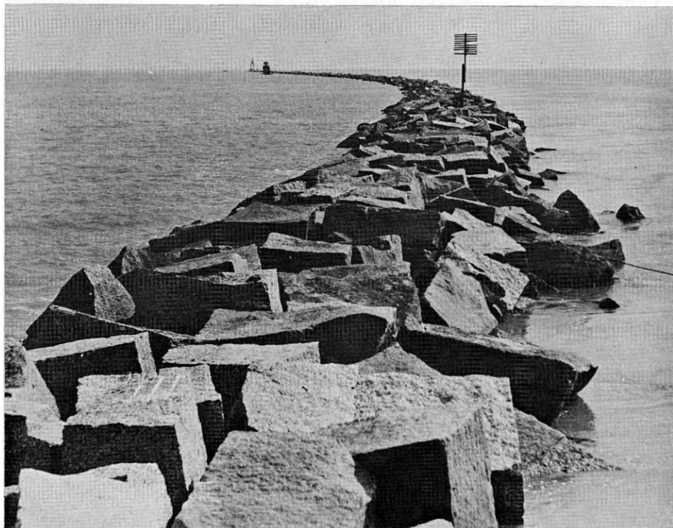
FIG. 4. Jetty at Galveston, Texas. Built with Precambrian granite blocks quarried and shipped from the Central Mineral Region (Pl. I). (Photograph by Corps of Engineers, U. S. Army, Galveston District, Galveston, Texas.)
