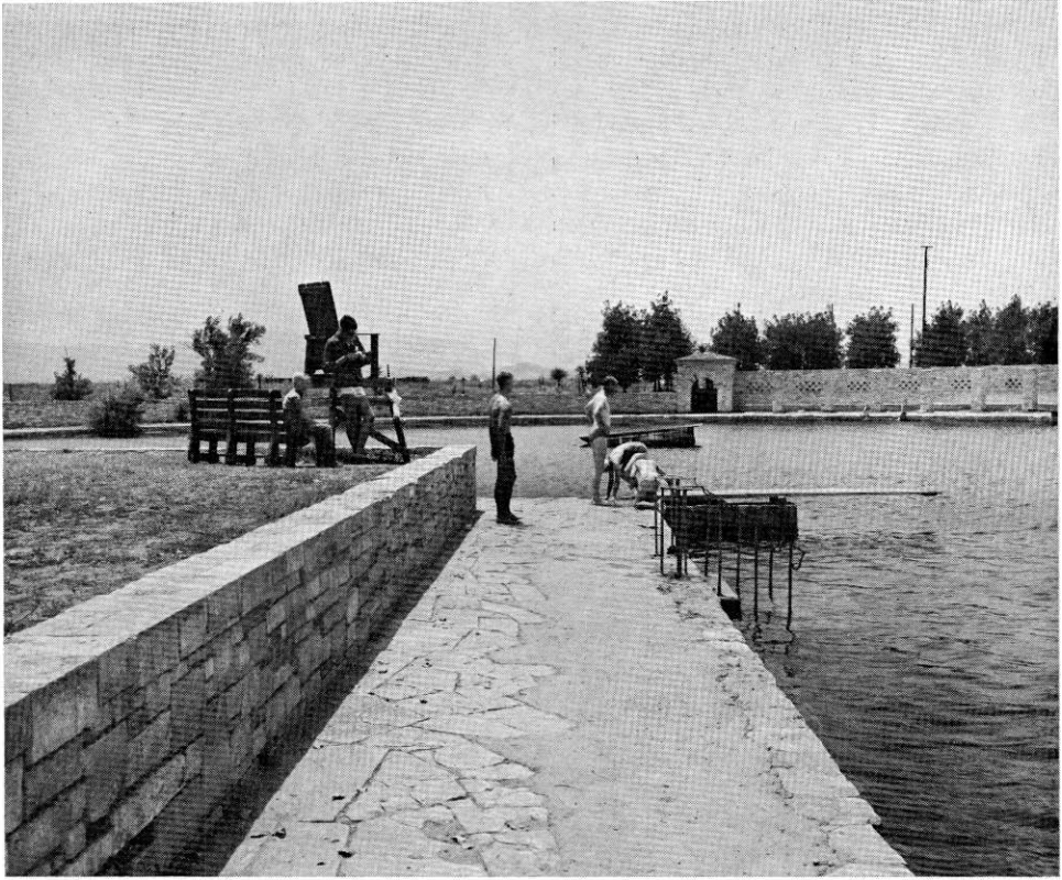
FIG. 25. The Balmorhea swimming pool which incorporates the total flow of San Solomon Spring. The spring was used by the Indians and frontiersmen and later for irrigation. Prior to the building of the masonry walls and walks of native Boquillas Flagstone, the water issued from a large swamp. (Photograph by Texas Parks and Wildlife Department.)
