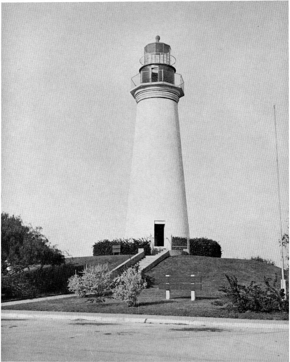
FIG. 93. Port Isabel Lighthouse. The only damage by Hurricane Beulah was four broken window panes. (Photograph by Texas Parks and Wildlife Department.)
