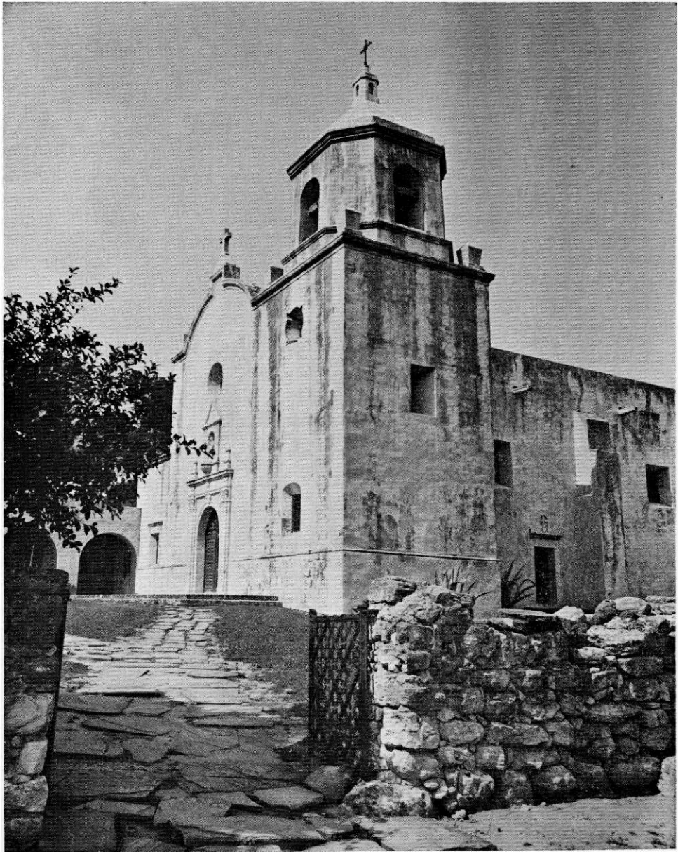
FIG. 63. Mission Señora del Espíritu Santo de Zúñiga at Goliad State Park. Stone in wall at gate to the mission is sandstone from the Goliad Formation. (Photograph by Texas Parks and Wildlife Department.)
