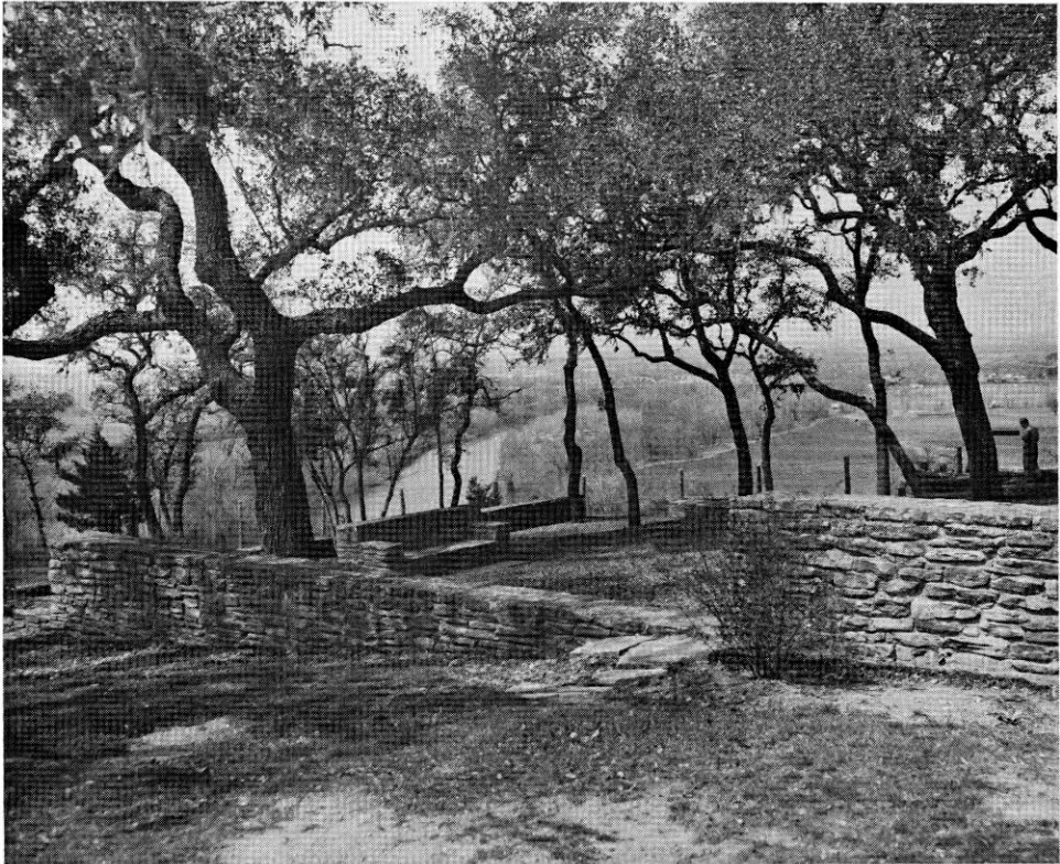
FIG. 78. Rest area at Monument Hill overlooking the terraced Colorado River valley. Outskirts of La Grange at upper right. Masonry wall constructed of Moulton Sandstone member of the Oakville Formation. Colorado River with cultivated terrace to right. (Photograph by Texas Parks and Wildlife Department.)
