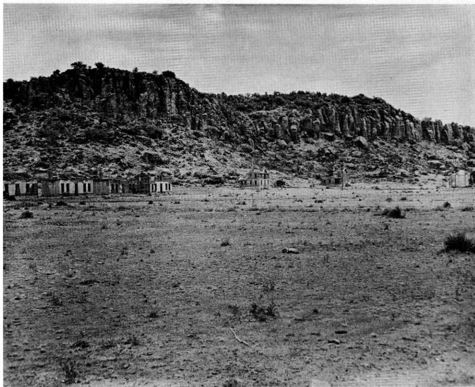
FIG. 44. Officers' Row at Old Fort Davis, 1854 to 1891. Following establishment of the National Historic Site (1963), these buildings along with others were reconstructed. During the 1860's and 1870's, Indian snipers shot arrows from crevices in the rhyolite cliff at rear. The palisades structure in the lava is due to weathering and erosion along joints in the Star Mountain rhyolite. (Photograph by Texas Parks and Wildlife Department.)
