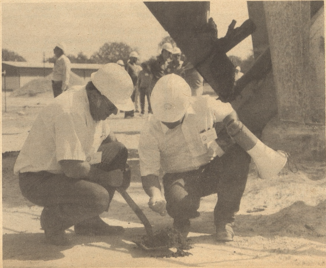
Instructor Lamar James, right, gives seminar participant Thomas Chapman some pointers on how to judge hot mix quality at a batch plant.
