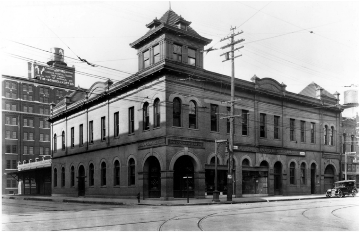
The St. Louis Southwestern Railway, popularly called the Cotton Belt, constructed this fine brick depot at the southwest corner of Commerce and Lamar. It opened in 1903 and survived until 1947.
