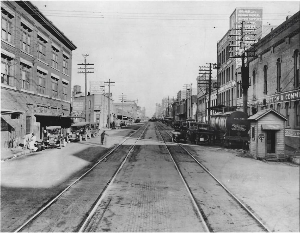
This view of Pacific Avenue clearly shows the railroad tracks running down the middle of the street, with brick pavers between the rails. The tracks were removed in 1923.
