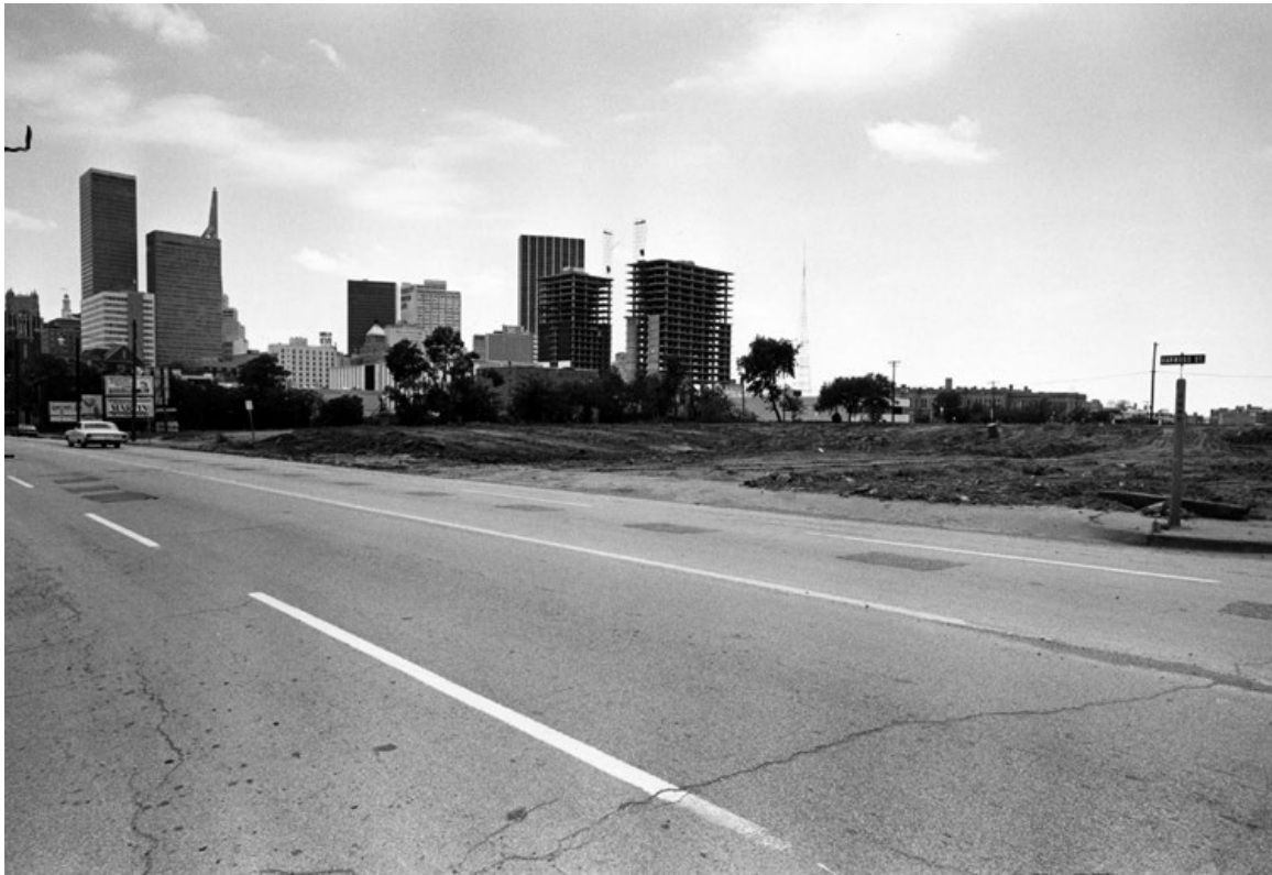
George Schrader was instrumental in re-designing Woodall Rodgers Freeway, connecting Central and Stemmons Expressways, below grade rather than as an elevated road. This photo shows Harwood Street with land being cleared to the west for excavation. This stretch of Harwood was later eliminated when Klyde Warren Park was constructed.
