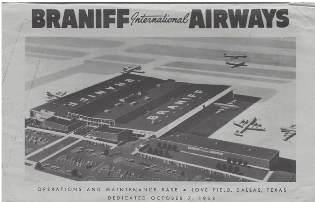
Braniff's $6.5 million Operation and Maintenance Base at Love Field opened in 1958 to make operations more efficient for maintaining its entire fleet.
