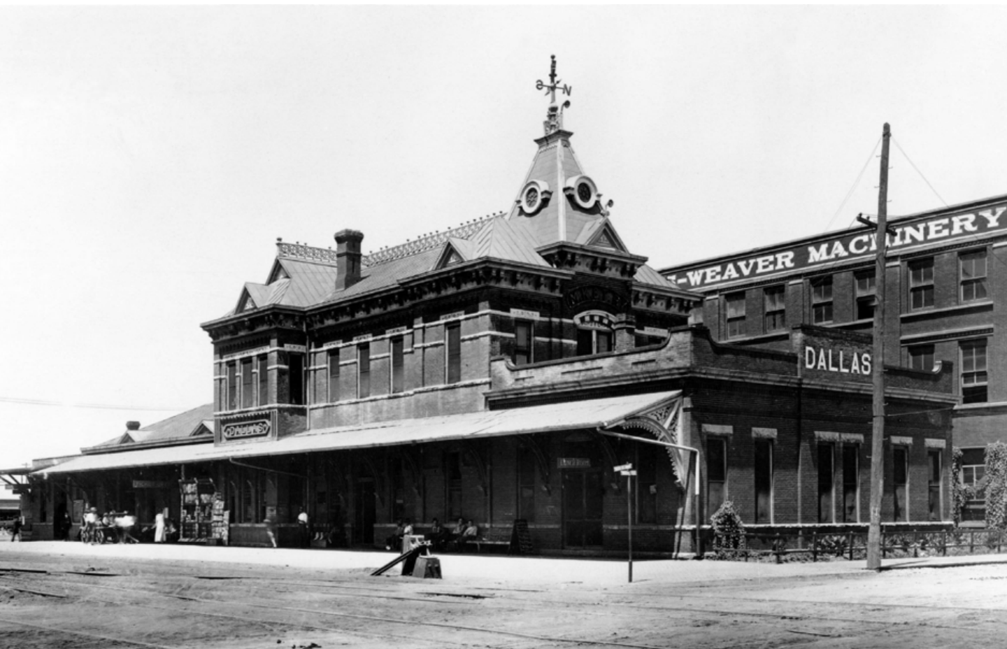
The Missouri-Kansas-Texas Railway (MKT) erected this handsome Second Empire-style depot at Pacific and Market streets in 1890. It survived until 1924.
