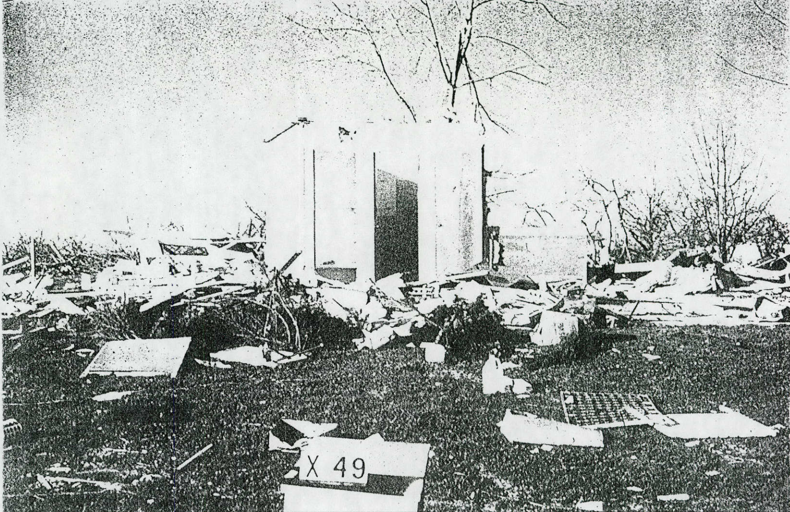
ABOVE: A STORM SHELTER THAT SURVIVED THE OKLAHOMA CITY TORNADO IN 1999.
