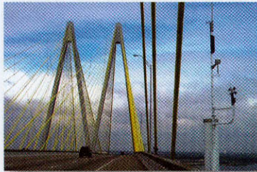
Weather station on the Fred Hartman Bridge, which spans the Houston Ship Channel.
