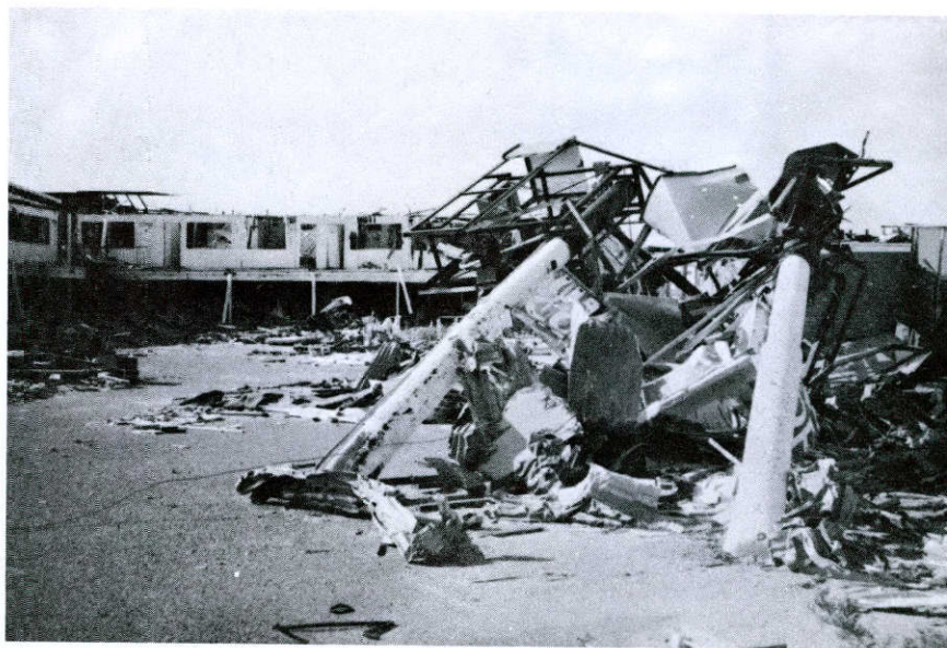
FIGURE 4. DAMAGE TO SIGN STRUCTURE AT RAMADA INN MOTOR HOTEL
