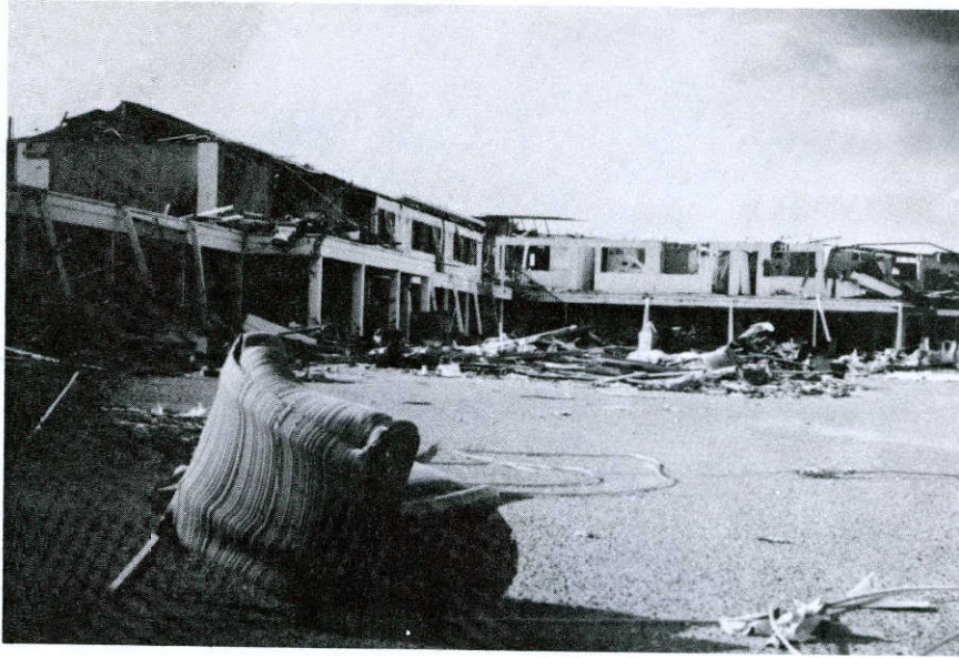
FIGURE 3. DESTRUCTION AT RAMADA INN MOTOR HOTEL
