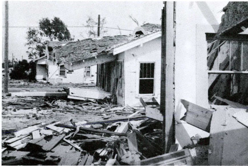
FIGURE 5. RESIDENTIAL DESTRUCTION ON 9th STREET NEAR AVENUE Q
