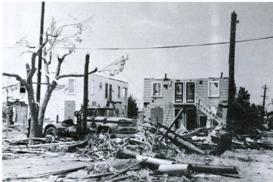
FIGURE 6. RESIDENTIAL DESTRUCTION ON 7th STREET NEAR AVENUE Q
