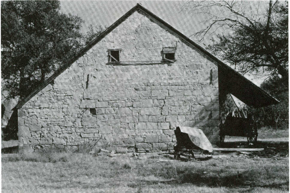
FIG. 4.—Typical Silesian Polish cottages showing the similarity of such structures in Poland and Texas. The upper structure is in the village of Centawa, Opole Voivodeship, and the lower structure, the Gawlik house built in 1858, is in Panna Maria. Note the steeply arched roofs designed to allow snow to slip off easily in the winter. Photographs by the author.
