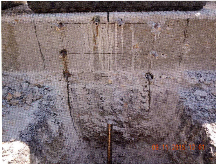
Figure 4.19 Joint condition before gage installation
