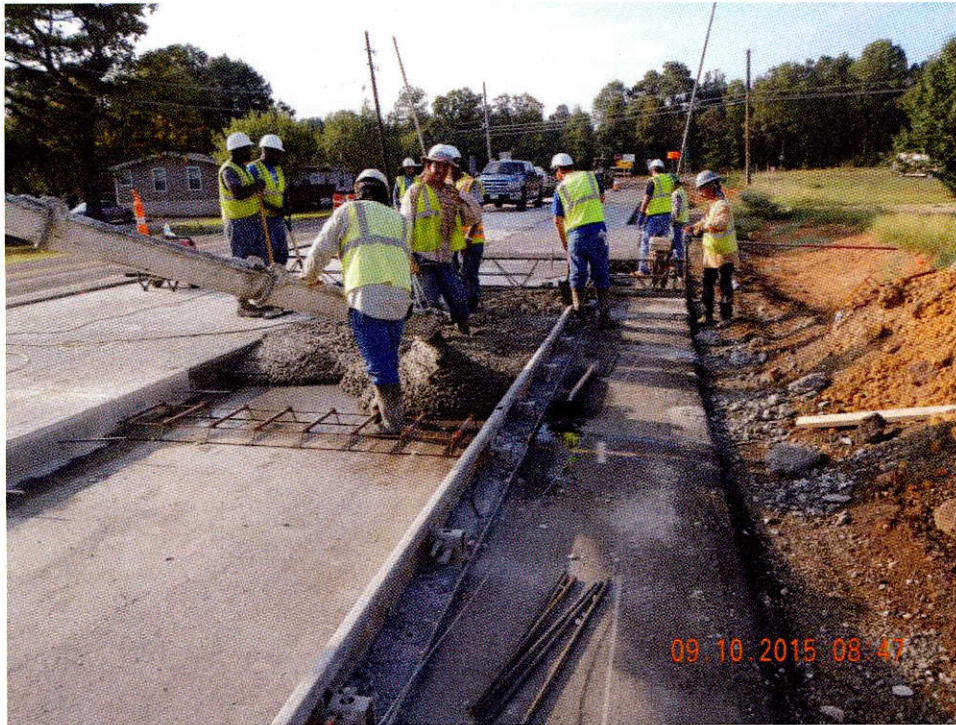
Figure 4.15 Concrete placement on FM 2253
