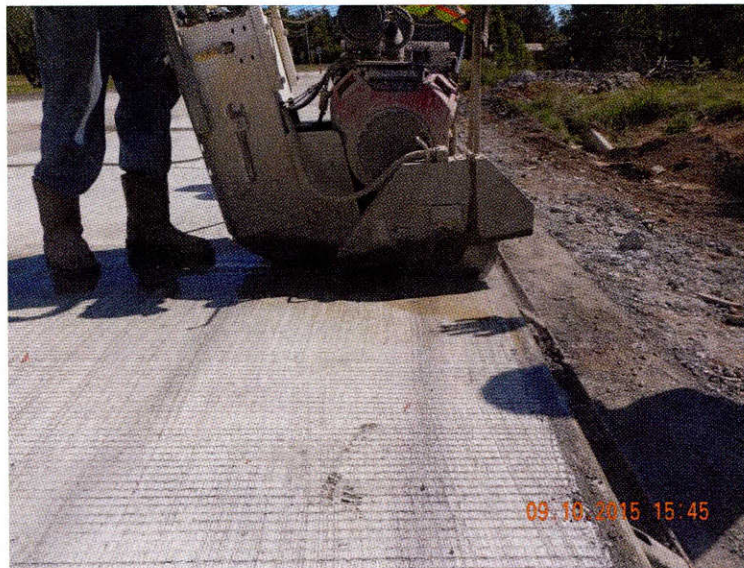
Figure 4.20 Sawcut at pavement edge
