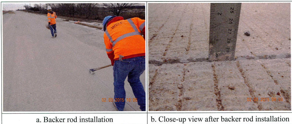
Figure 2.8 Backer rod installation
