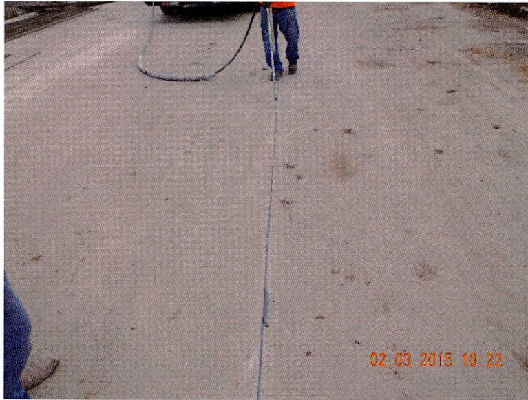
Figure 2.9 Sealant installation
