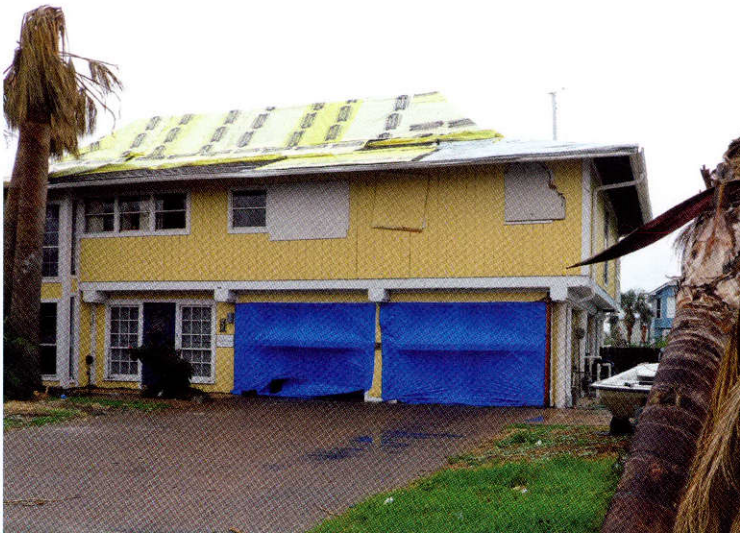
Garage doors are often the first part of a house to suffer wind damage, as seen on the Key Allegro home on the left. On the right, Texas Sea Grant Senior Associate Director for Planning and Extension and CRC Co-Director Heather Wade photographs a much sturdier one at a house near Salt Lake during the FEMA Mitigation Assessment Team's damage survey.
