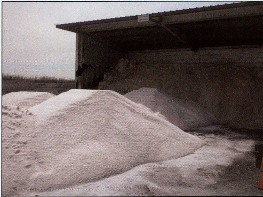
FIG 30. Granular (solid) chemicals should be stored inside to prevent runoff of salts dissolved by precipitation
