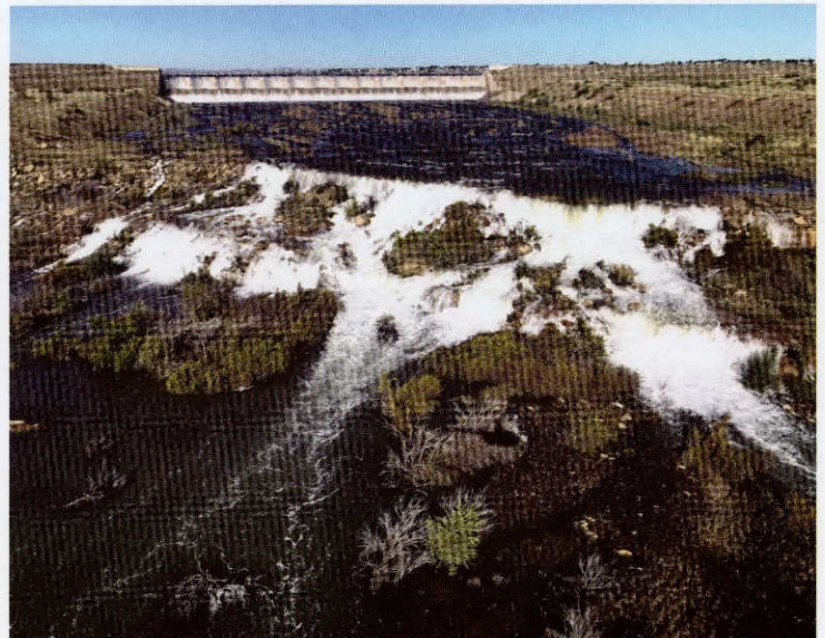
Ute Lake spillway on October 8, 2017. Picture courtesy of Kent Satterwhite.
