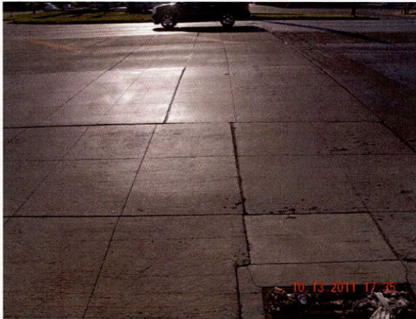
Figure 4.3 Differential Slab Displacements at Longitudinal Joints in Midland
