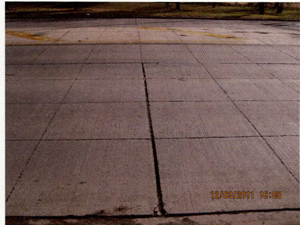
Figure 4.4 Differential Slab Displacements at Longitudinal Joints in Abilene
