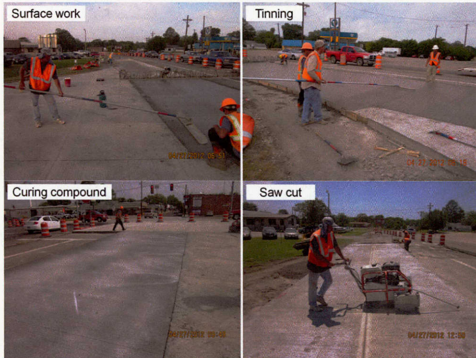
(b) Finishing and saw cut
