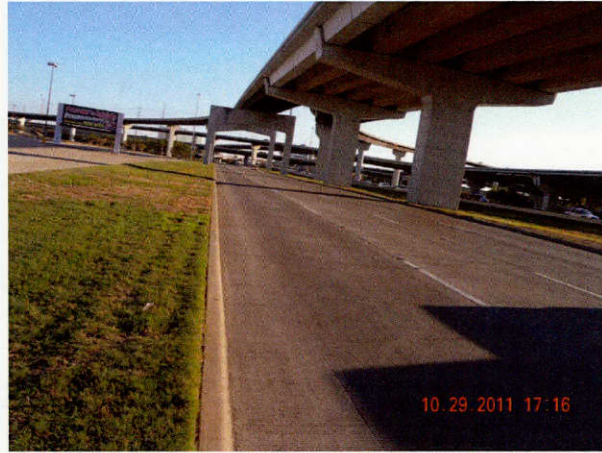
Figure 4.2 Excellent Performance of Fast-Track Concrete Pavement Built In 1993
