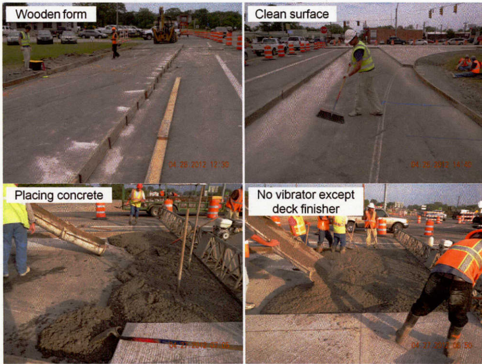
(A) Surface Preparation and Concrete Placement
