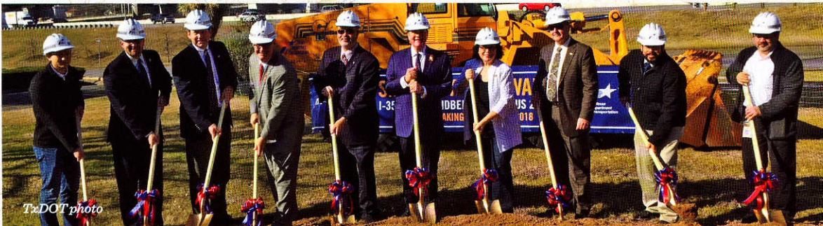
State and local officials break ground on the I-35 project from Rundberg Lane to U.S. 290 East.
