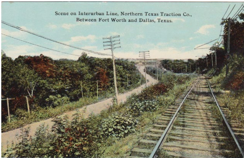
This image of the interurban tracks between Fort Worth and Dallas shows the electric lines on the right that powered the trains. The dirt country lane on the left would soon attract more automobiles, providing competition to the interurban.
