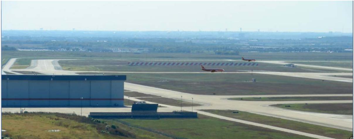
Figure 42: View from East ATCT to SE EAT
