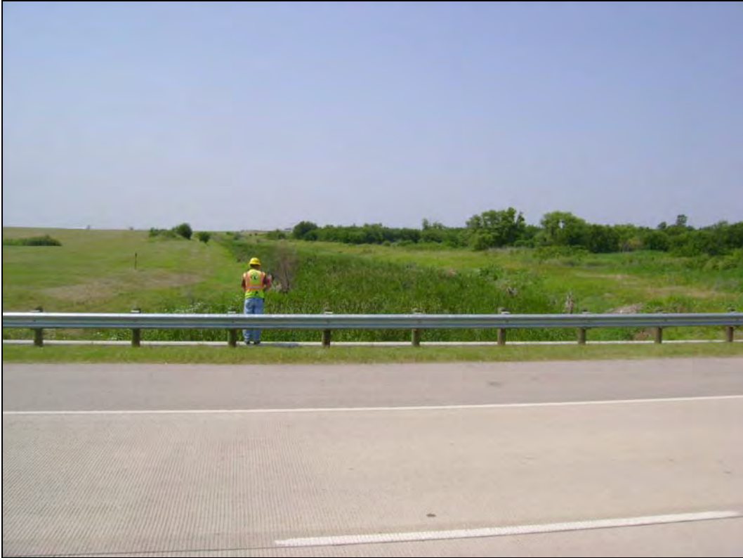
Figure 2. Looking South from the culvert at Airfield Drive.
