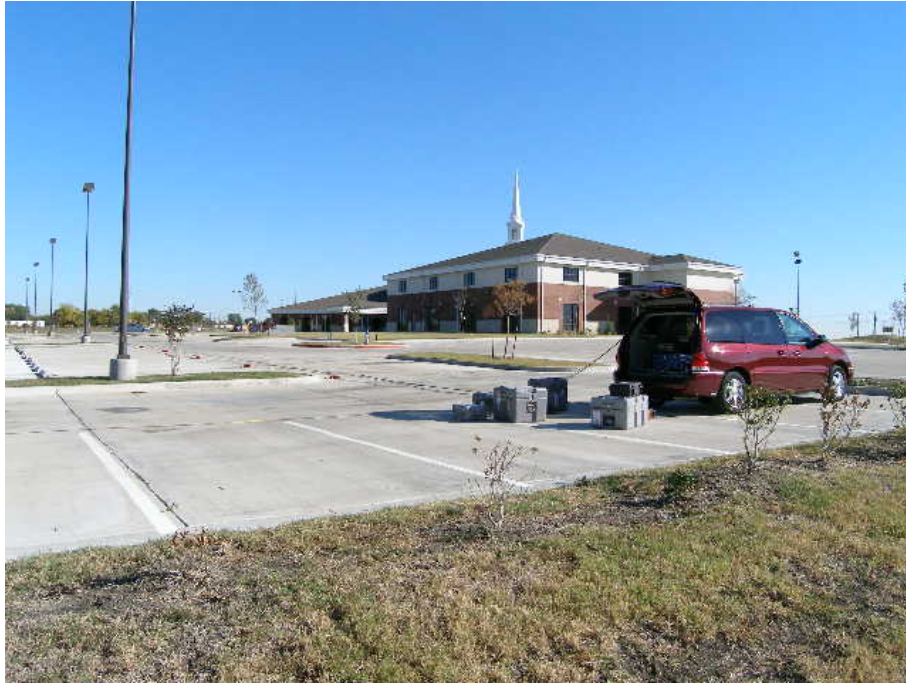
Figure A-6. Site V-1, Mt. Hebron Baptist Church, Garland
