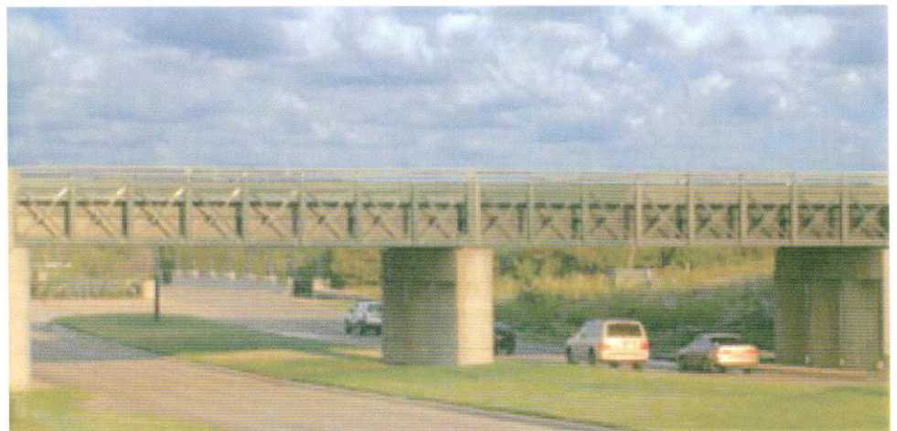
Steel Thru Girder Bridge Example
