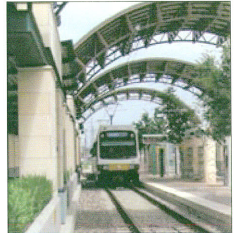
DART Light Rail at Downtown Garland Station
