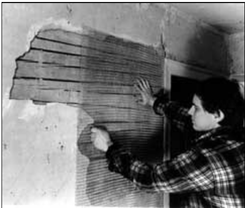
In this New Hampshire residence dating from the 1790s, the original plaster was a single coat of lime, sand, and horsehair applied over split lath. A one-coat repair, in this case, is appropriate. Photo: John Leeke.
