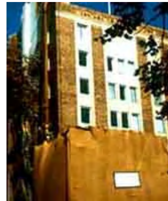
The lower floors of this historic brick and architectural terra-cotta building have been covered during chemical cleaning to protect pedestrians and vehicular traffic from potentially harmful overspray. Photo: NPS files.
