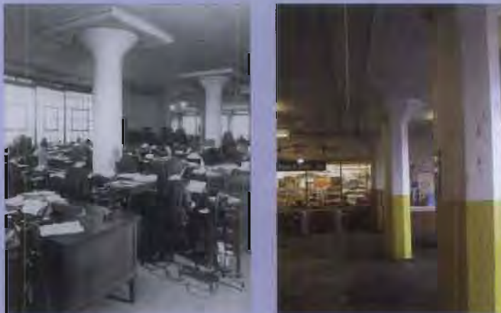
Figure 11. Whether in a circa 1925 office (left) or in a parking garage and retail facility (right), exposed concrete structures help characterize these building interiors. Photo: Minnesota Historical Society (left).
