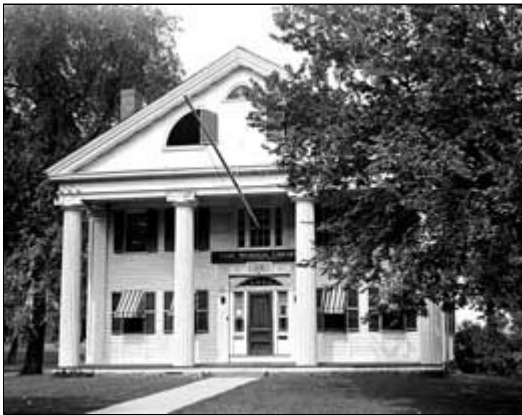
This 19th c. building in Massachusetts employed several energy-conserving features in its historic design, including shade trees, roof overhangs, awnings and shutters. Photo: HABS collection, NPS.
