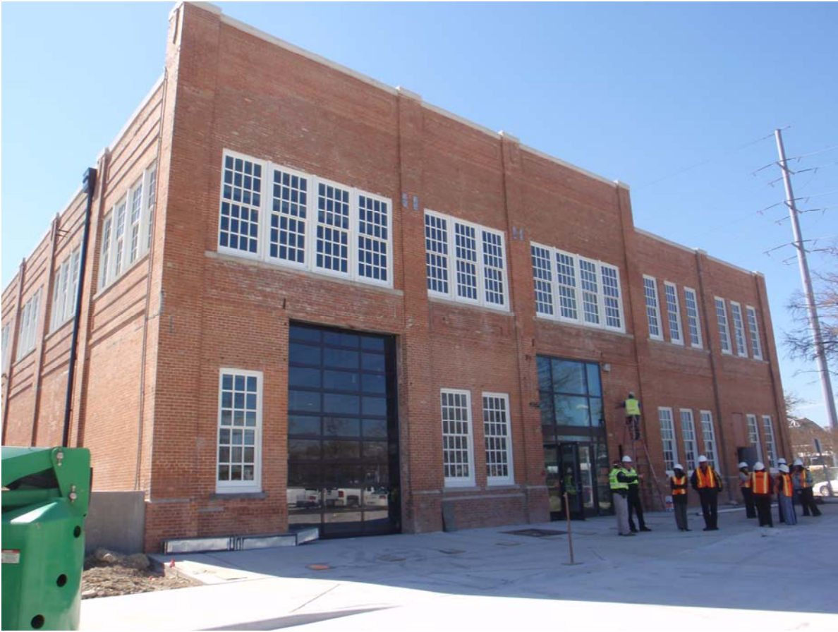
Figure 10: Replacement steel windows on north facade
