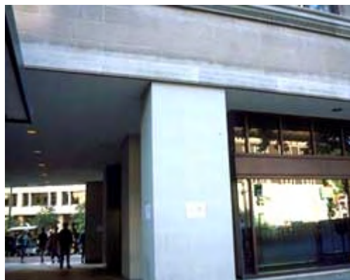
The difference in color between the bottom and the top of the stone spandrel is the only clue to the presence of a clear barrier coating. Photo: NPS files.
