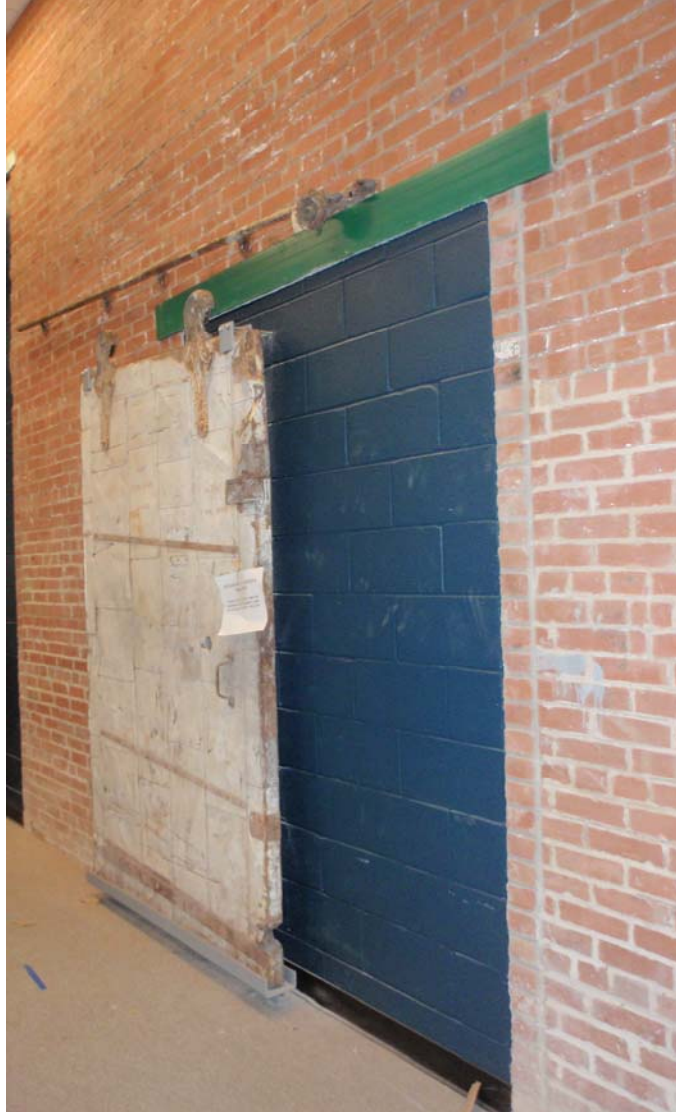
Figure 5: Fire Door and Mechanism reinstalled
