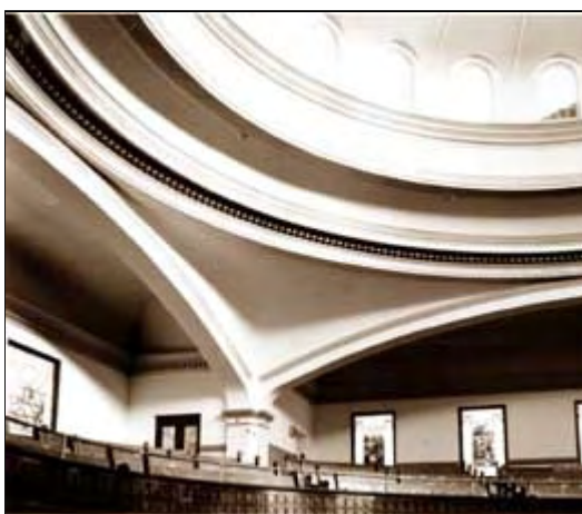
Plaster was used as the interior surface
