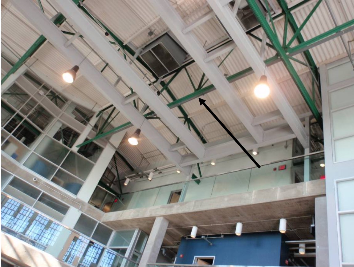
Figure 23: Historic trusses (painted green)
