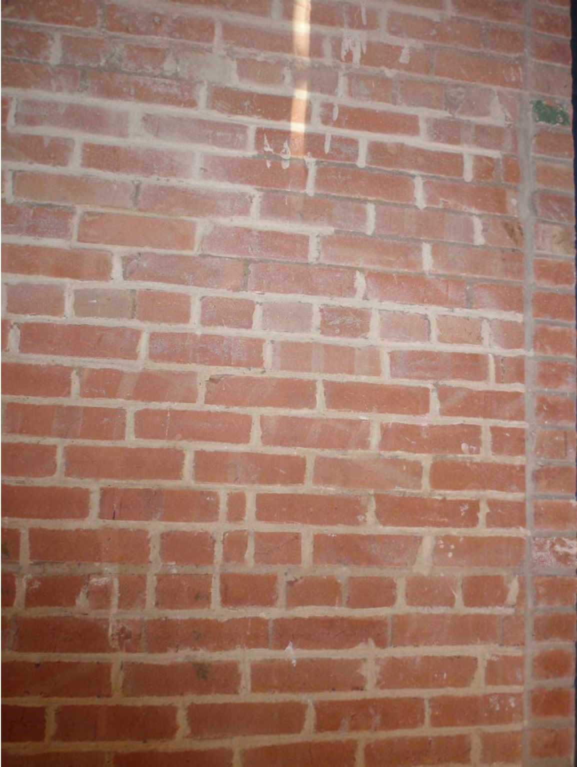
Figure 7: Masonry after cleaning and repointing.
