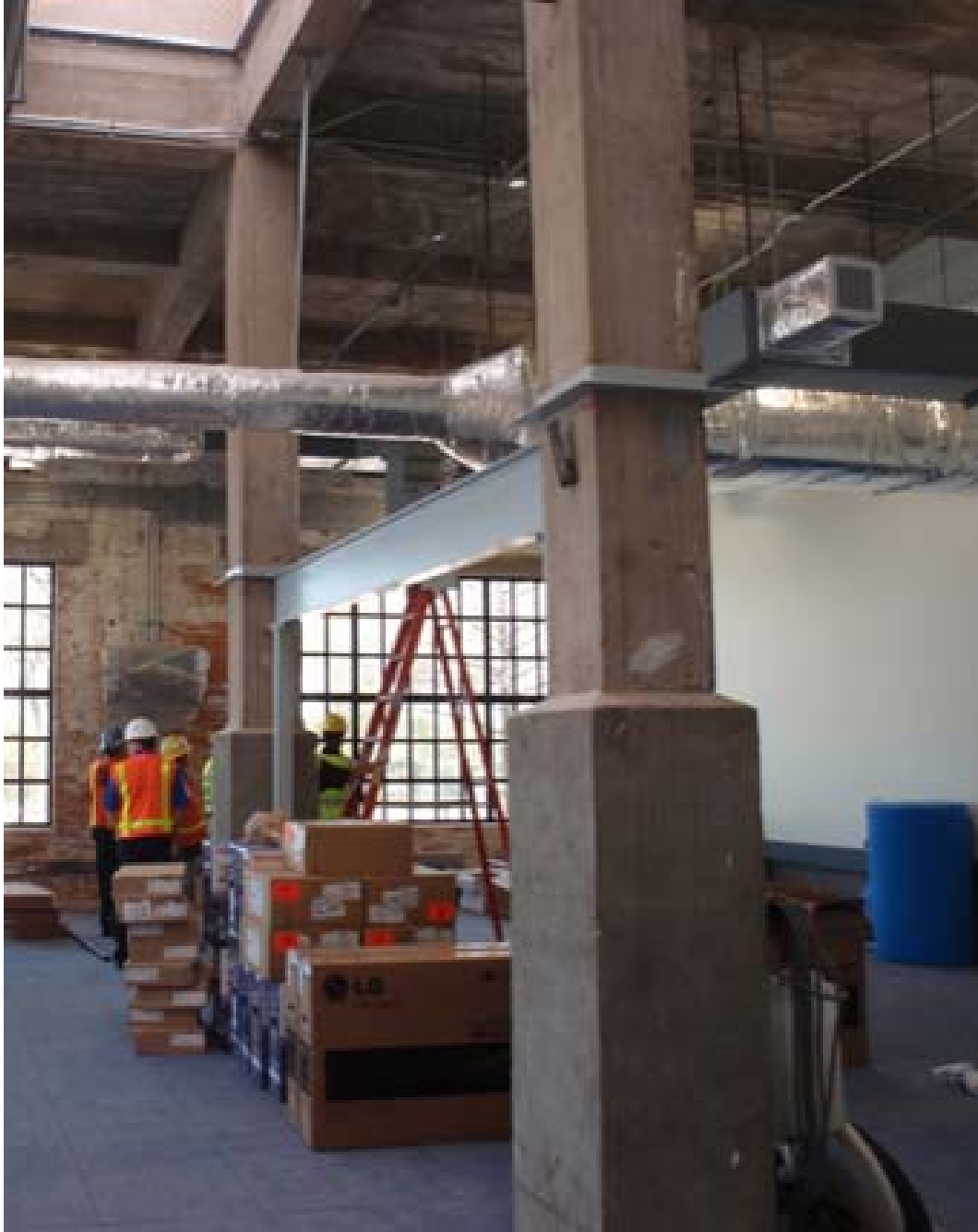
Figure 17: Columns after cleaning
