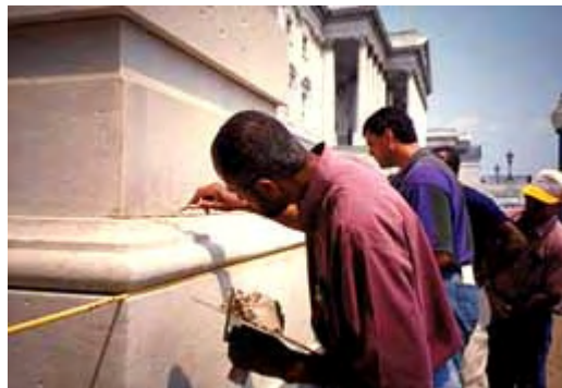
Masons practice using lime putty mortar to repair historic marble. Photo: NPS files.
