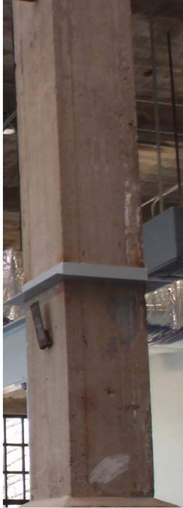
Figure 18: Close-up of historic concrete column
