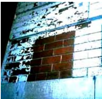
Any cleaning method should be tested before using it on historic masonry. Photo: NPS files.
