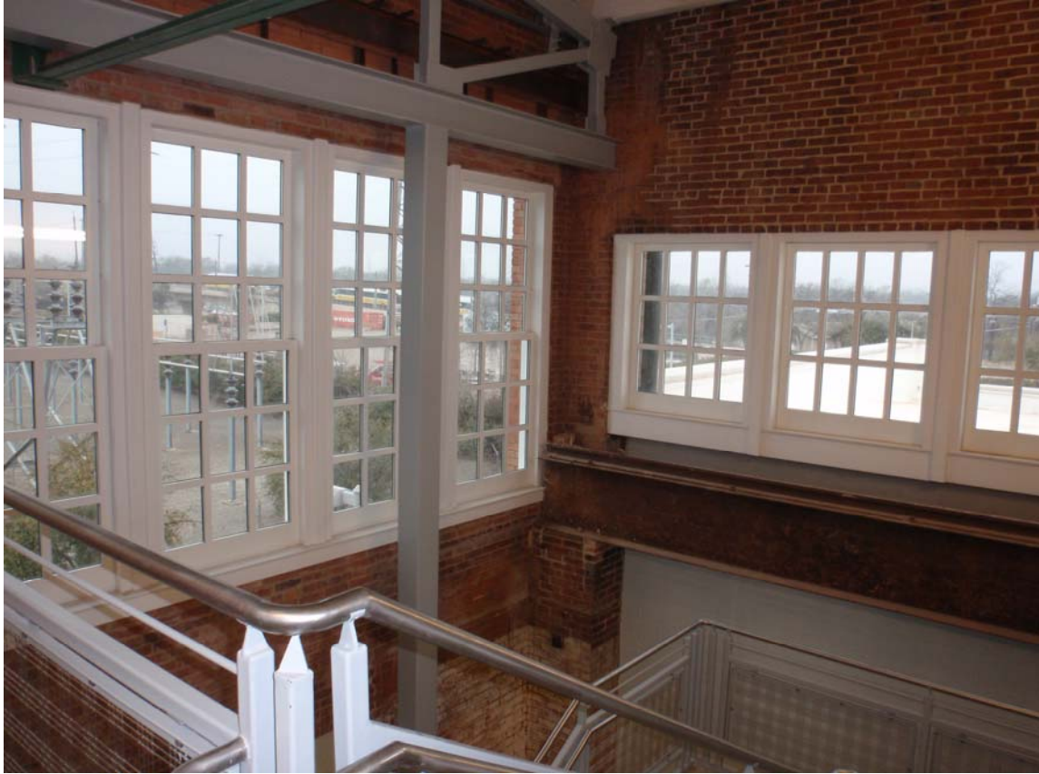
Figure 11: New interior wood window sills and surrounds
