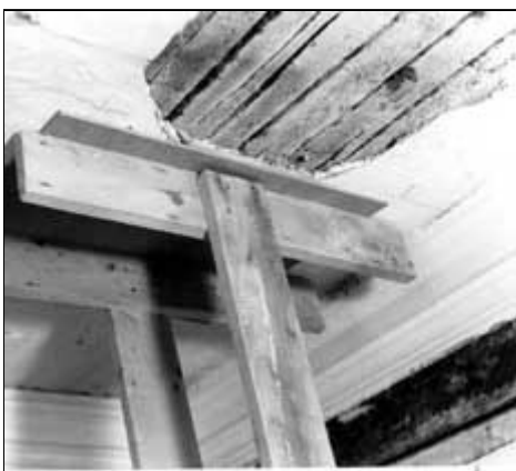
When ceiling repairs are made with wet plaster or with an injected adhesive mixture, the old loose plaster must be supported with a plywood brace until re-keying is complete. Photo: John Leeke.
