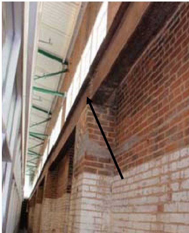
Figure 22: Crane Rail Support Beam (arrow)
