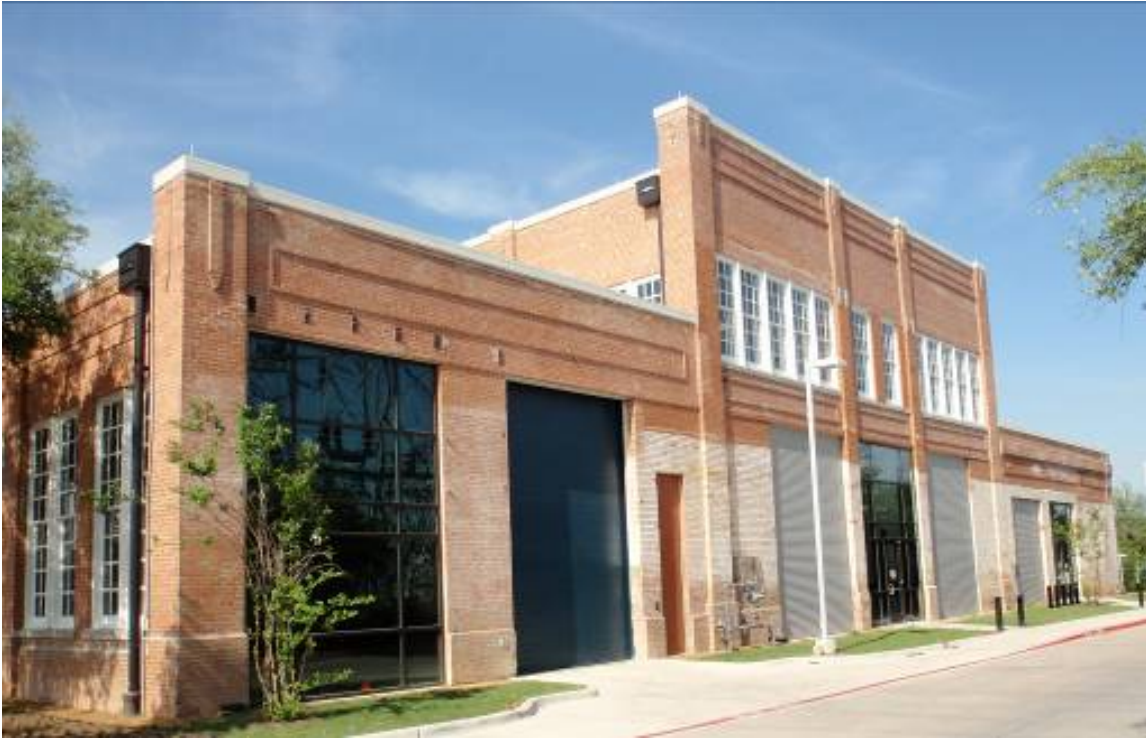
Figure 12: South façade with historic openings
