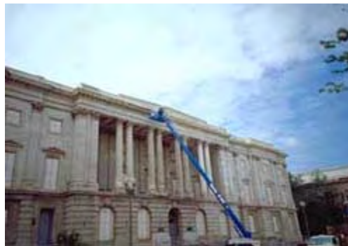
Low-to-medium-pressure steam (hot-pressurized water washing) is a gentle method of softening heavy soiling deposits and cleaning historic marble. Photo: NPS files.
