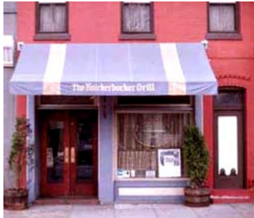
Awnings reduce heat gain in the summer and, when they are raised in the winter, radiant heat from the sun provides free supplementary heat. Photo: NPS files.
