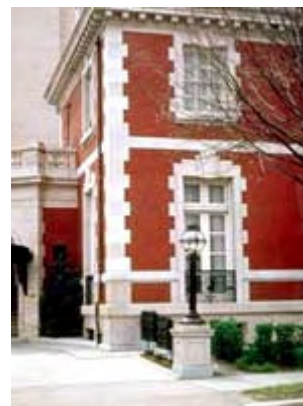
The decorative trim on this brick building is architectural terra-cotta intended to simulate the limestone foundation. Photo: NPS files.
