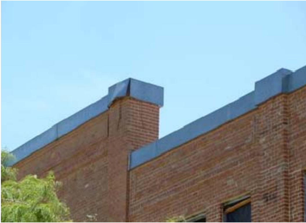
Figure 15: Parapet Cap during repair
