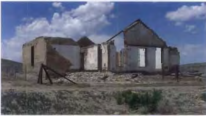
Figure 2. Chatterton House was the home of the post trader at Fort Fred Steel in Wyoming, one of several forts established in the 1860s to protect the Union Pacific Railroad. The walls of the post trader's house were built using stone aggregate and lime, without cement. The use of this material presents special preservation challenges.
