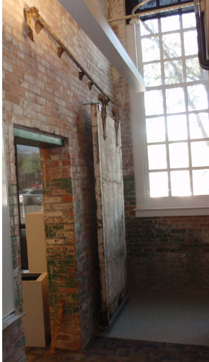
Figure 6: Fire Door reinstalled
