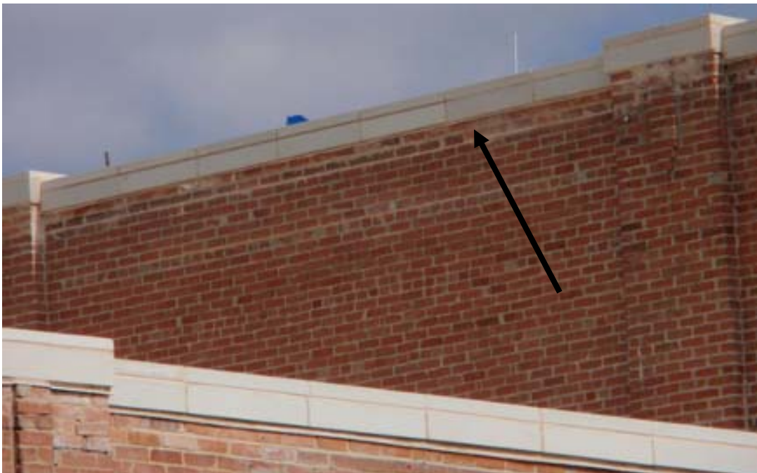
Figure 16: Parapet Cap after repair
