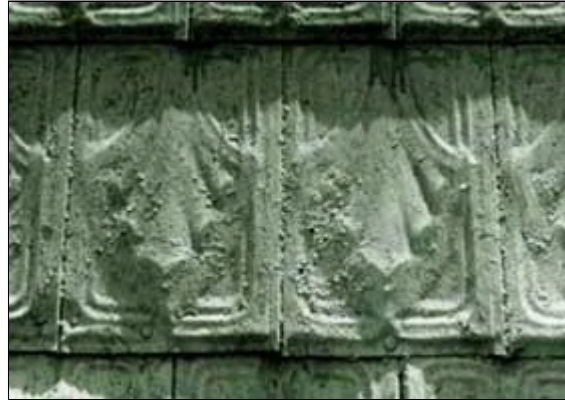
Tin shingles, commonly embossed to imitate wood or tile, or with a decorative design, were popular as an inexpensive, textured roofing material. Photo: NPS files.
