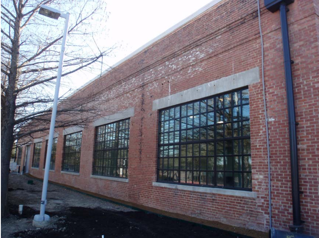
Figure 9: Replacement steel windows on east facade
