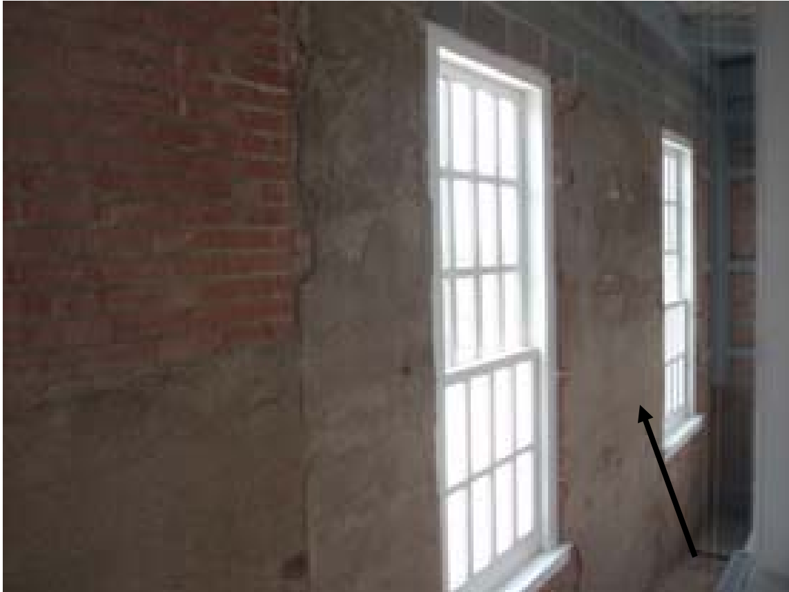
Figure 25: Historic plaster (arrow) on second floor
