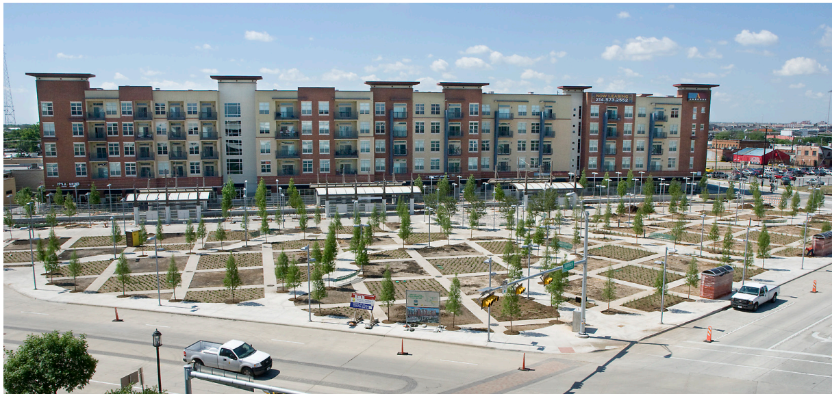
Baylor University Medical Center Station with new Ambrose development
