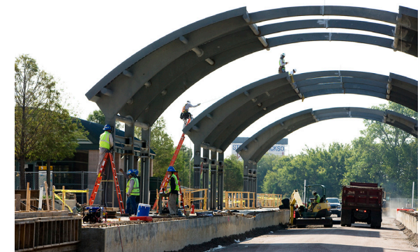
Lake June Station construction
