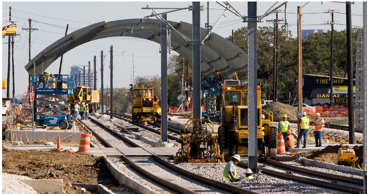
Love Field Station construction
