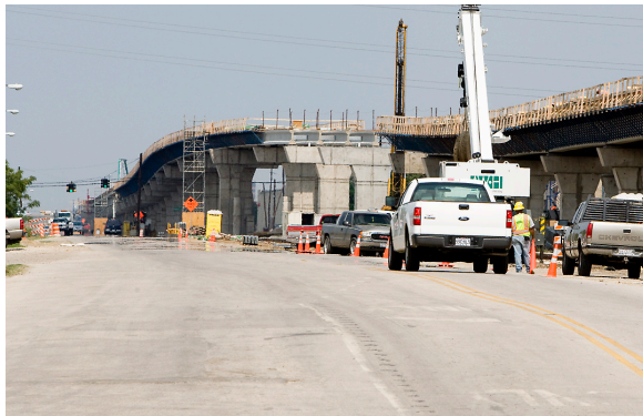
Construction of aerial structure at Walnut Hill Lane
