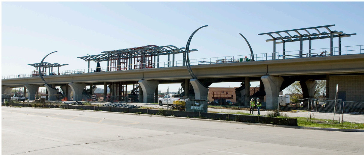
Inwood Station construction
